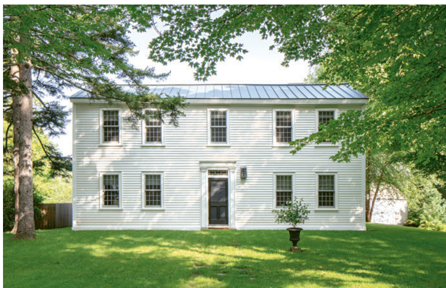
The Federal-style house had been added onto multiple times in its 200-plus years, but only the original portion was salvageable. A revised set of additions follows the path of the old while blazing new trails.
