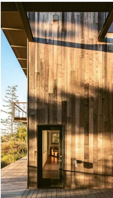
This page: The house floats above the site's thick and thorny vegetation like a seafaring vessel. The steel-framed dogtrot, fitted with only a partial roof, helps bring much-needed light into the great room. Thermally treated ash cladding and decking, applied in random lengths, resists the maritime climate.
