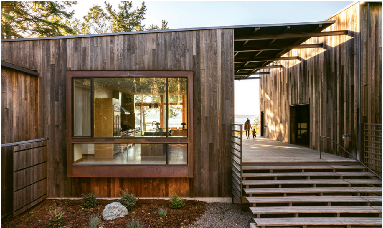
Just a small corner of this island parcel was buildable, with many restrictions on construction near the bluff. So architect Dan Shipley's design splits the plan in two and cantilevers portions to protect vegetation and catch scarce sunlight, and tips roofs to shed rainwater away from the shoreline.
