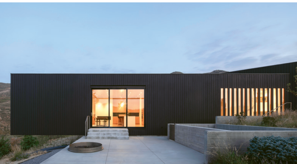
This page: The house's cantilevered volumes nestle below the ridgeline, preserving views from the road. Outdoor living is clustered in patios that also serve as fire breaks. A blackened steel firepit warms cool nights, and a board-formed concrete dog run protects the family pet from predators.
