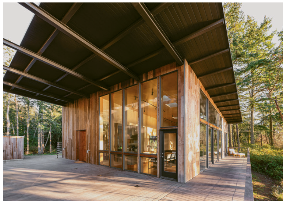
This page: The house floats above the site's thick and thorny vegetation like a seafaring vessel. The steel-framed dogtrot, fitted with only a partial roof, helps bring much-needed light into the great room. Thermally treated ash cladding and decking, applied in random lengths, resists the maritime climate.
