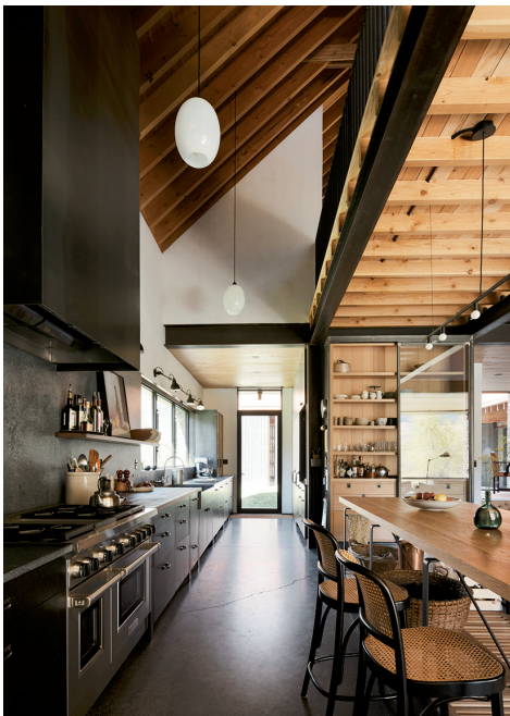
This page: The open kitchen reveals the sturdy structure of the house, fortified by steel for seismic loads. Faced in board-formed concrete, an Argentinian wood-fired grill anchors one end of the cooking wall. Soapstone counters top the ebonized wood cabinets, and Douglas fir paneling clads the ceilings. Concrete floors are geothermal radiant.
