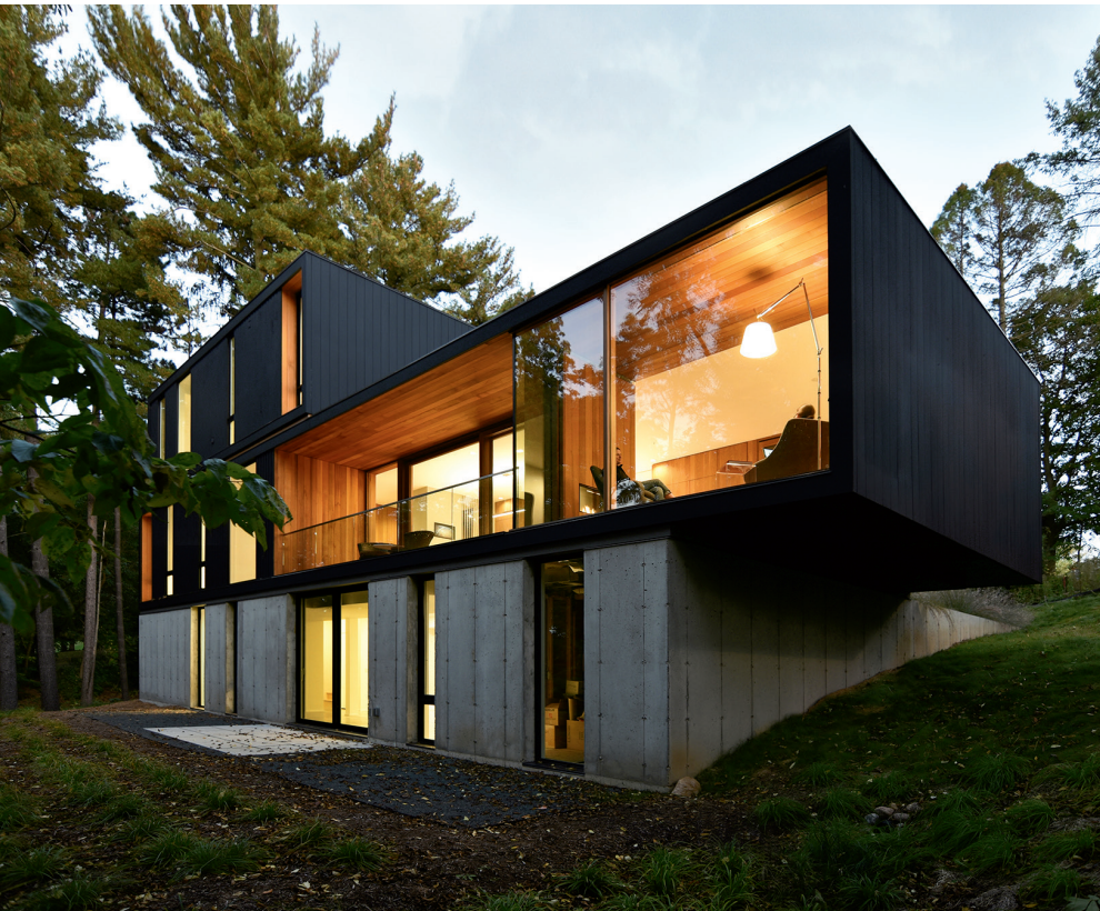
The firm's stacked boxes facilitate cantilevers over site imperfections. Here, the blunt ends of the boxes employ flat-applied siding, while the broad sides are either glazed or beveled lap siding.
