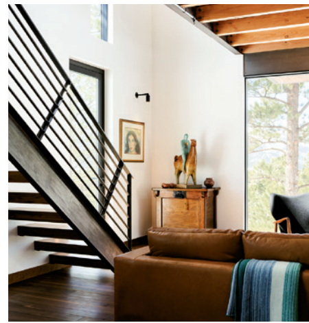
This page and opposite: Carbon steel grating sheds snow and provides secure footing on the path to the front door, which is sheltered by the overhanging bedroom suite. Inside, 8½-foot-tall window modules make the house feel larger than it is, and exposed metal and wood framing minimizes material use, in keeping with the owner’s philosophy of simple living. The black-painted sprinkler system recedes into the steel framing.
