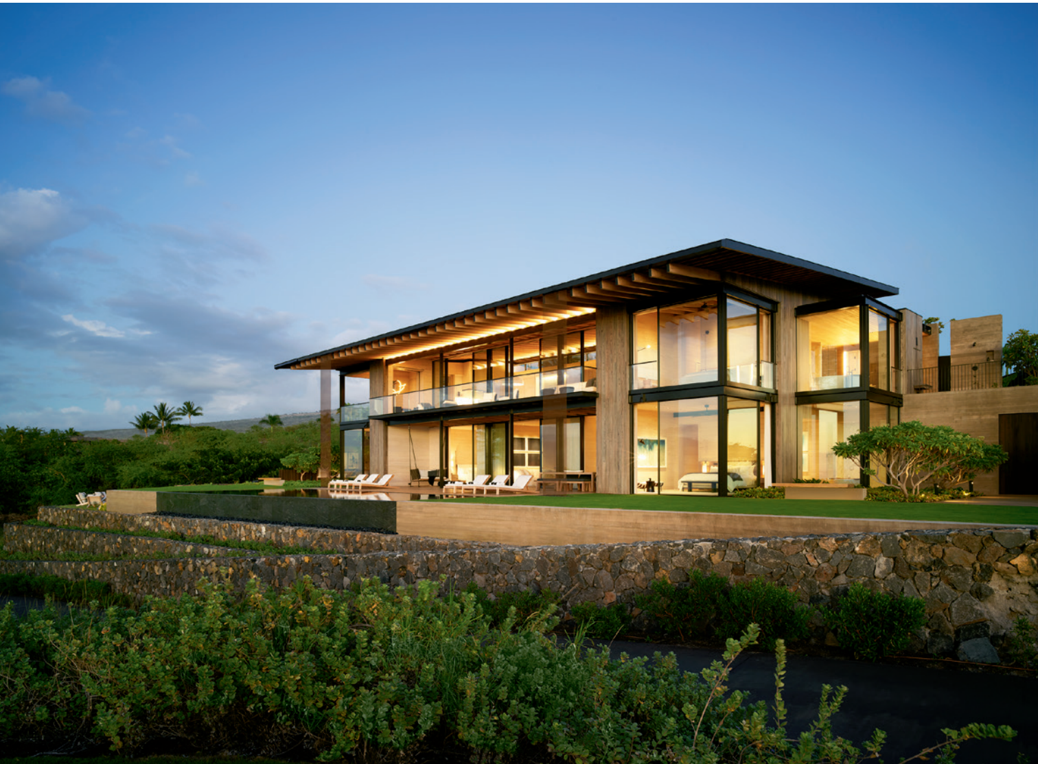
This page: Architect Greg Warner, who grew up in Hawaii, points out that local residents have always built their properties up on plinths. “It was a simple way to create a level area.” For the design team, the plinth and basalt retaining walls solved the problem of the lot’s steep grade down to the water. The cant of the landscaping resulted in a dynamic wedge-shaped, disappearing-edge pool.
