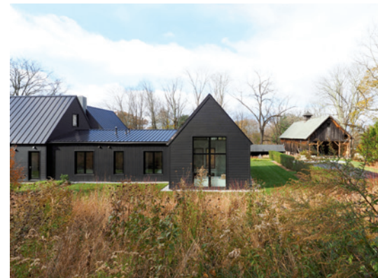
This page: A new second home in upstate New York takes its design cues from two restored barns on the property, echoing their combination of high- and low-gabled forms.
