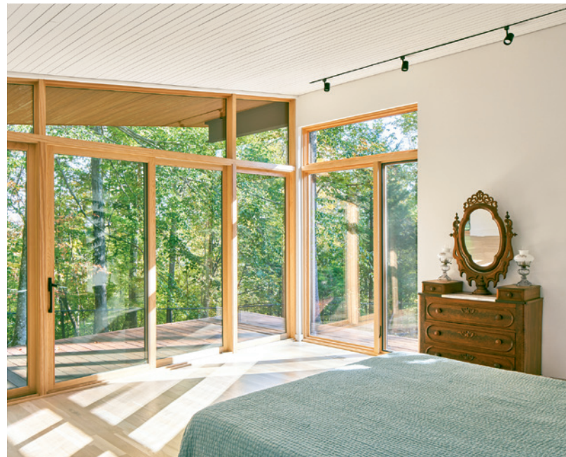
Large-format windows were not in the budget, so the architects specified 8-foot-tall units and topped them with transoms to accomplish the effect of more generous openings.
