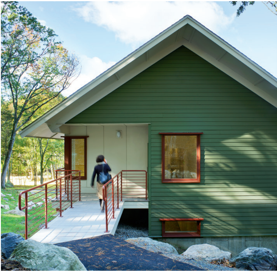
Previous and this page: For this private school dormitory project, Eck MacNeely Architects applied knowledge gained as residential architects to problem solve. The firm rotated the building on the steeply sloped site, giving it access to the campus at high and low points and increasing its daylighting.
