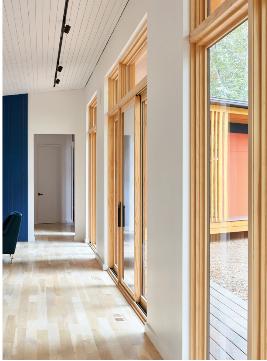
Large-format windows were not in the budget, so the architects specified 8-foot-tall units and topped them with transoms to accomplish the effect of more generous openings.
