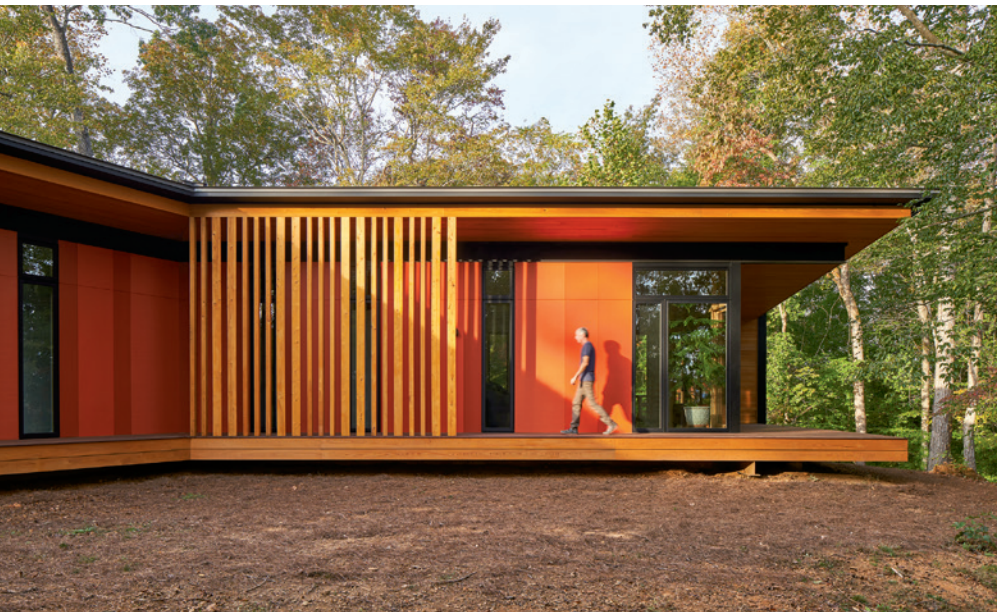
Exterior materials aim for low maintenance—metal roof and cladding, cementitious panels, cumaru decking, and cypress screening, soffits, fascia, and skirt boards. The cypress screening, reinforced with metal from behind, provides a measure of privacy for the primary bedroom. Exterior colors mimic the forest’s fall tapestry of hues.
