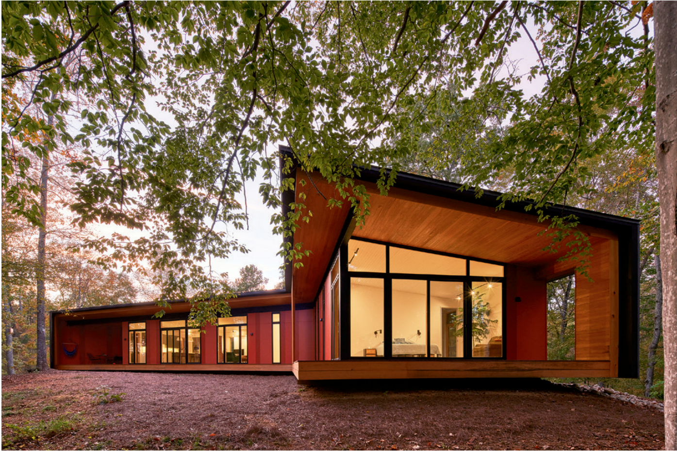
Exterior materials aim for low maintenance—metal roof and cladding, cementitious panels, cumaru decking, and cypress screening, soffits, fascia, and skirt boards. The cypress screening, reinforced with metal from behind, provides a measure of privacy for the primary bedroom. Exterior colors mimic the forest’s fall tapestry of hues.
