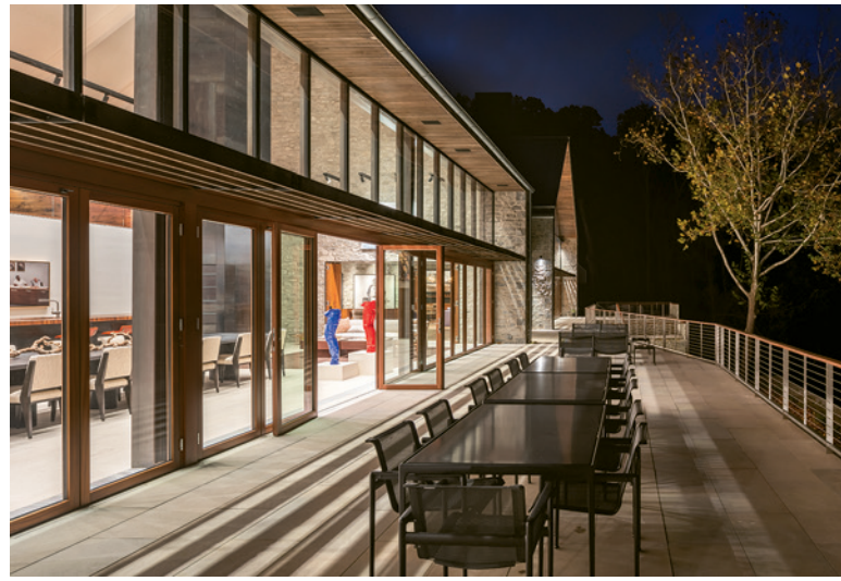
Window walls and terraces lead guests to the home's strongest features, the river and waterfall that once powered the mill. By day, there's the drama of the view; after dark, the water music claims center stage.
