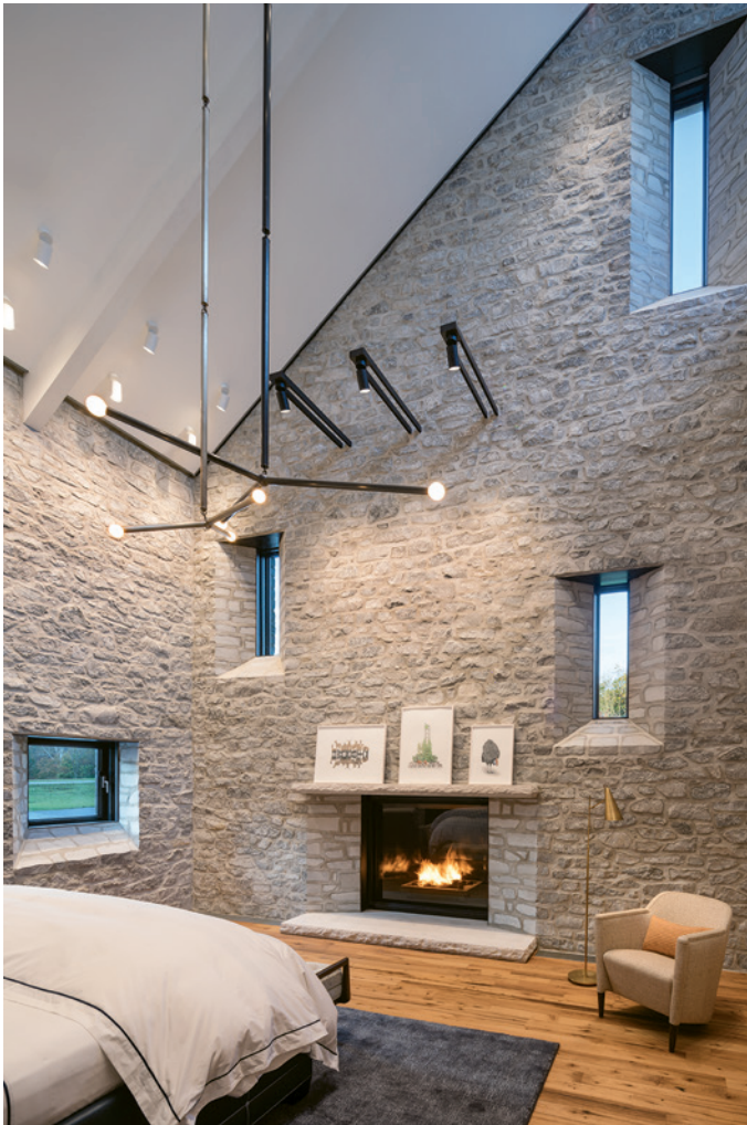
Above: Slotted windows in the main bedroom evoke old barns, where slants of light move across the floor during the course of the day. Instead of a simple veneer, the architects specified C-grade and had it installed 5 inches thick on exterior and interior walls, with a 12-inch layer of insulation in between. Below: A guest room on the mezzanine level of the family wing has its own balcony.
