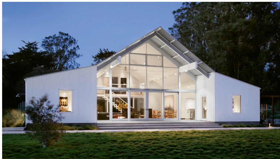
This page: TGH designed this modern barn house to engage its 160-acre site devoted to sustainable farming. Bedrooms and kitchen flank the lofty living room, opening to the long view south. Passive cooling and heating, thermal mass, plus geothermal and radiant systems earned it LEED Platinum.
