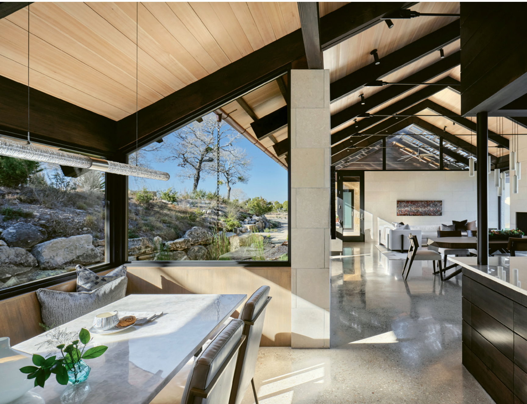
This page: In the great room, dark-stained framing contrasts with honed limestone walls and terrazzo-like concrete floors. The specks of color in the floor come from the Medina river rock aggregate used in the pour. Ceilings are hemlock with a transparent white glaze to preserve the evenness of the finish.
