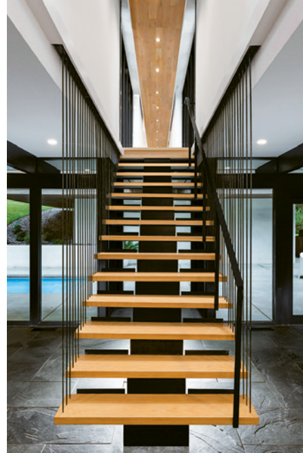
This page: The stair is entirely suspended from cables, but structure was added to comply with riser codes and to keep it from “swinging.” The home’s color palette derives from the original yellow walls and black beams.
