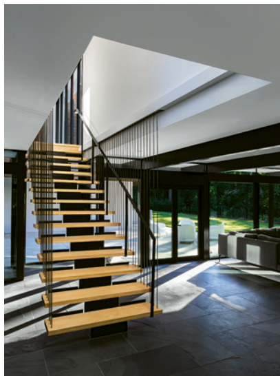
This page: The stair is entirely suspended from cables, but structure was added to comply with riser codes and to keep it from “swinging.” The home’s color palette derives from the original yellow walls and black beams.
