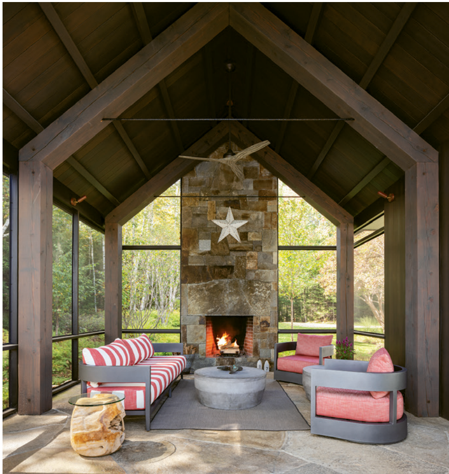
The timber-framed screened porch celebrates natural materials but conceals the hefty joinery required to support the weighty structure. Beams are joined by mortise and tenon connections, but hardware is hidden and only slim collar ties catch the eye.
