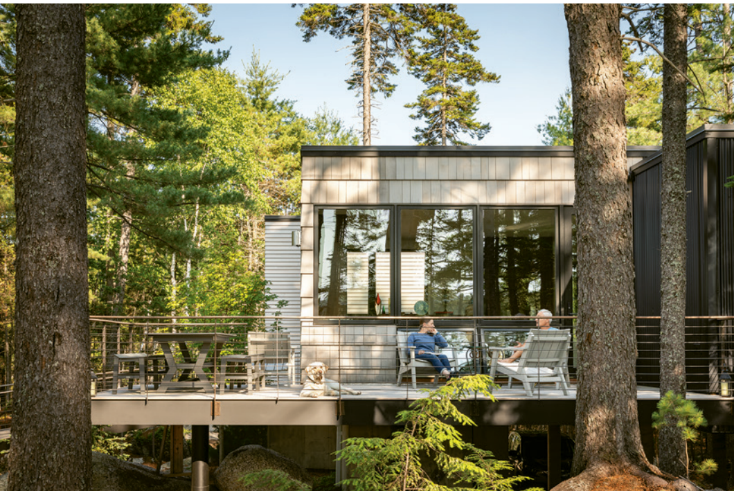
Cedar shingles are upsized for a more modern look and placed on a rainscreen for longevity. Long-wearing steel siding receives a contrasting, dark Kynar coating that suggests charred wood.
