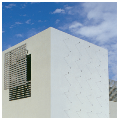
Steel leaves projecting on rods from the wall of Sunlit House cast shadows as the sun moves through its daily cycles and seasons.
