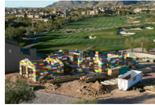
Left to right: The Special Olympics benefit build under construction and what the home will look like when its LEGO-like ICFs are covered in stucco.
