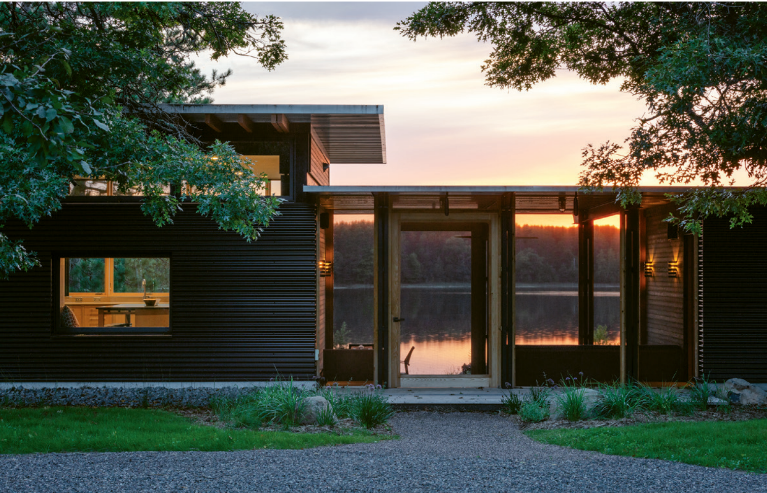
Black corrugated siding on the front elevation traces a shadowy frame for the glistening lake view.
