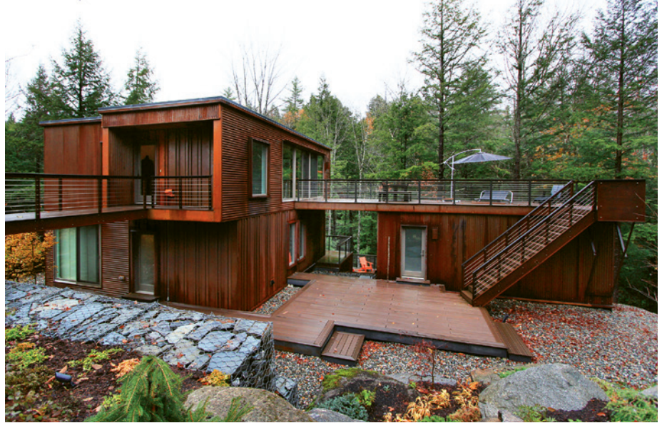
The clients for the Rocky Brook weeHouse in New Hampshire were repeat customers. Modules stack and pull apart from each other to climb the hilly creekside site and bathe in its natural setting.
