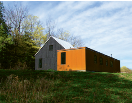
The Corning, N.Y., weebarnHouse is part weeHouse, part barnHouse, plus a garage shed. It combines modular and panelized construction, demonstrating the possibilities of mixing the firm's whole kit of parts.
