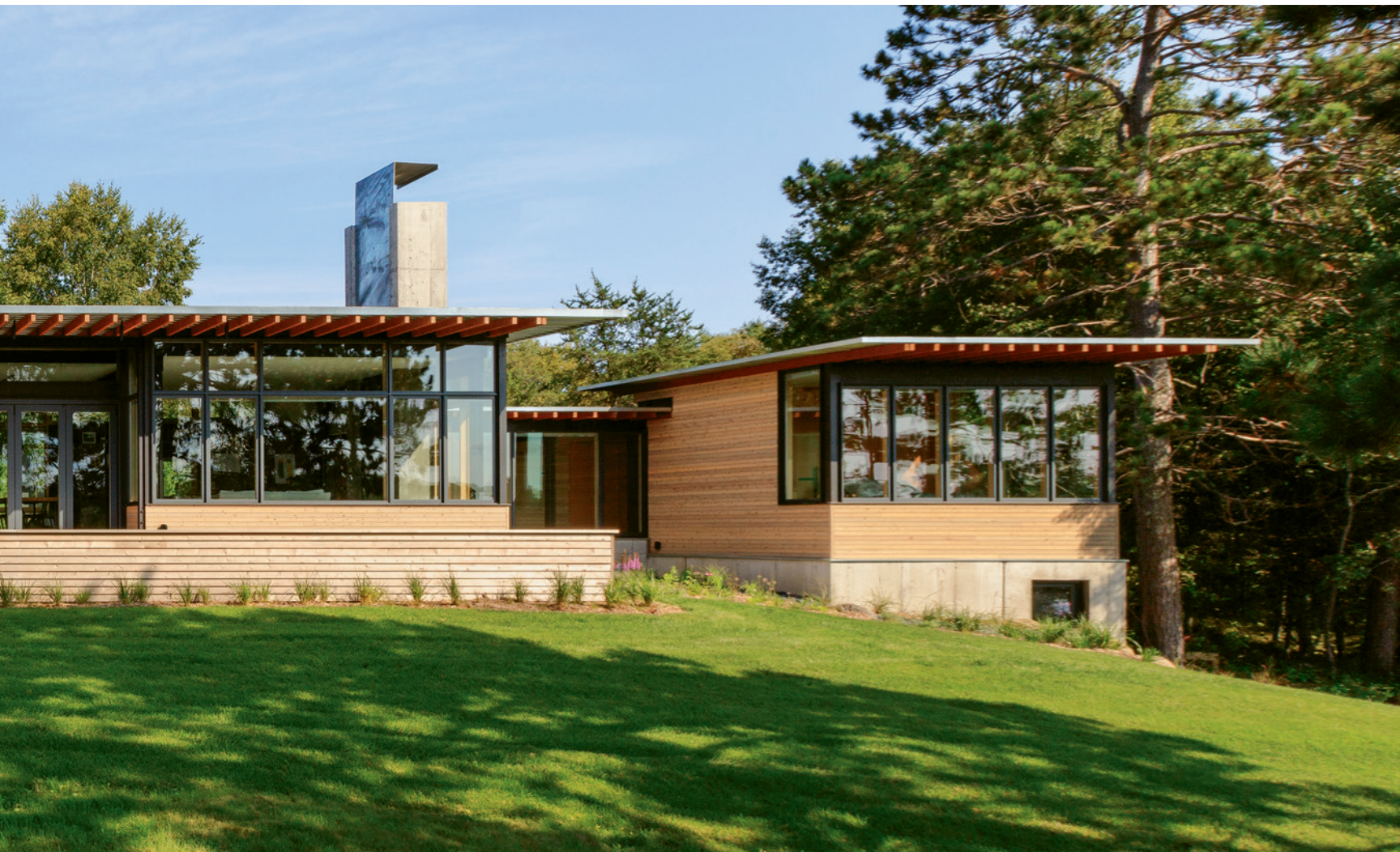
This page and opposite: The wide, one-story plan places “night boxes” (bedrooms) at the north and south ends, with the day box (kitchen, living, dining) in the center. The fireplace’s steel surround pierces the roof to become the chimney cap.
