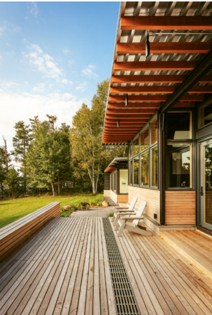
This page: The best views of the lake are westerly, requiring deep overhangs to shade interior spaces from afternoon glare. Hidden steel beams ensure the roof can support seasonal snow loads.
