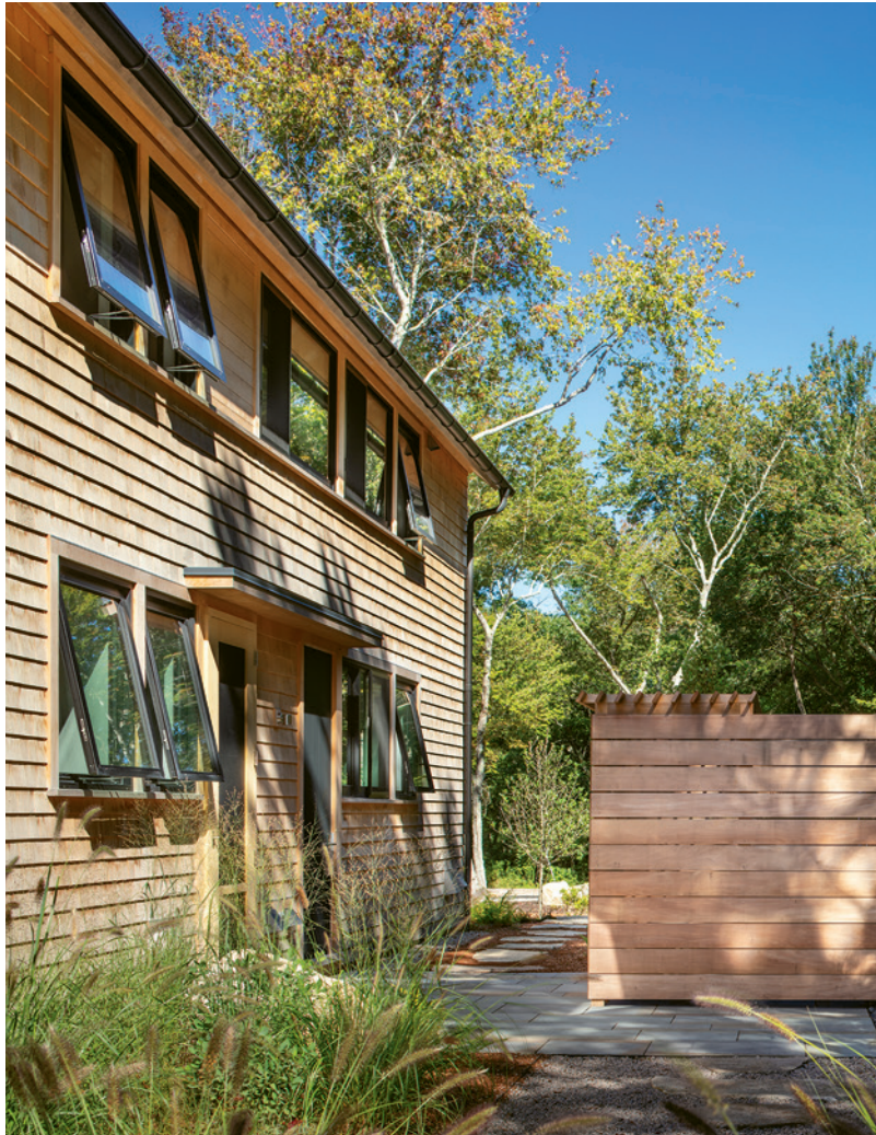
This page: Awning windows allow natural ventilation—even during summer downpours. An outdoor shower and adjacent mudroom place cleanup facilities near beach and pond activities, instead of the usual spot by the motor court.
