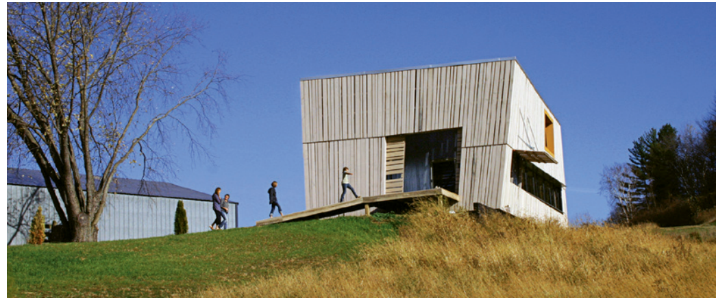
Photos: Courtesy Alchemy Architects
