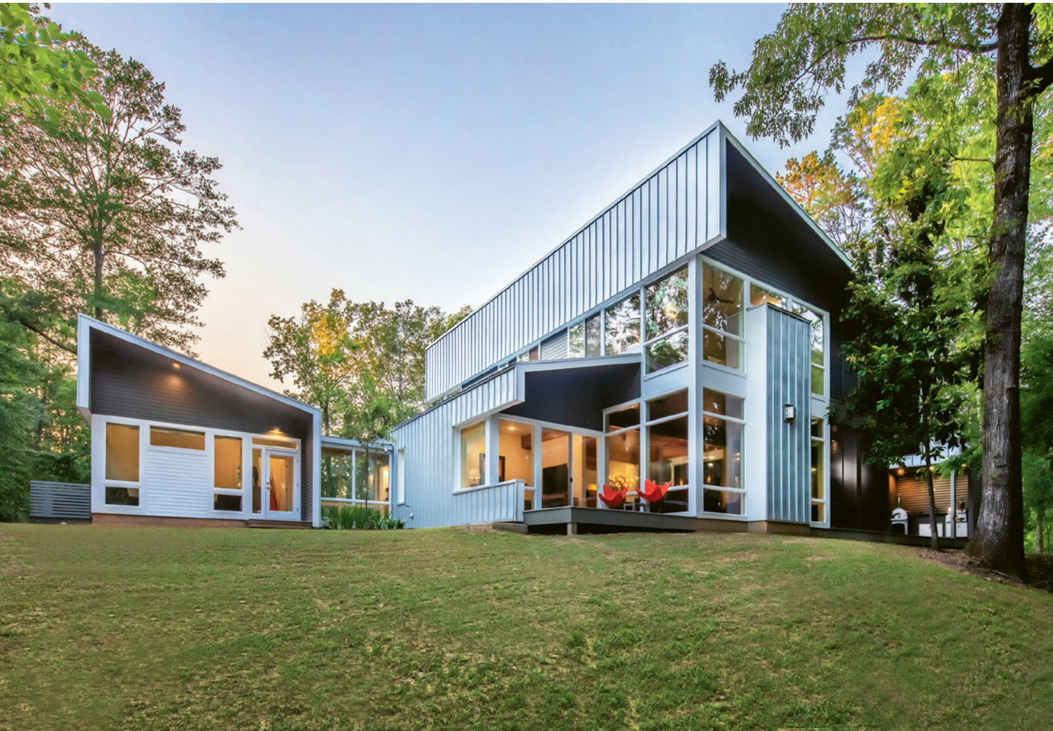
The dramatic folding roofs are cut away for windows to the view, but project past the walls to shelter openings from frequent downpours. Green cement siding recedes into the forested landscape.
