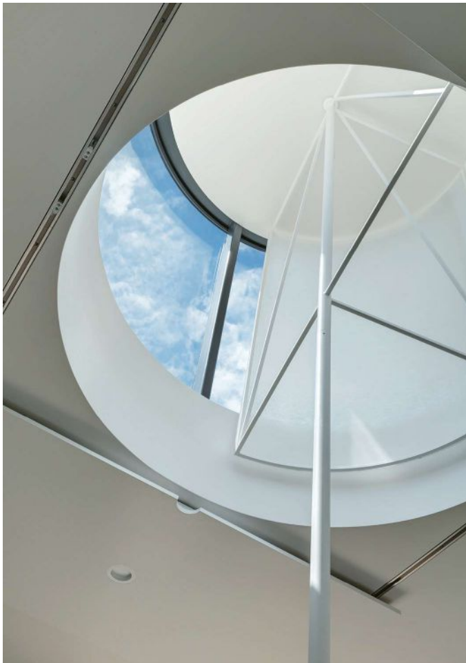
Clockwise from below left: Max's design is deferential to the original, but asserts its own subtle flourishes, including a series of roof monitors with manually operable Lumasite sails that open to fresh air and light. The bedrooms are wrapped in aluminum plates, sanded and screwed to a waterproof substrate.
