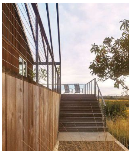
This page: Board-and-batten siding is a staple material of farm buildings, but here it's given a modern tweak in the crispness of its detailing and its juxtaposition with sections of flat vertical siding.
