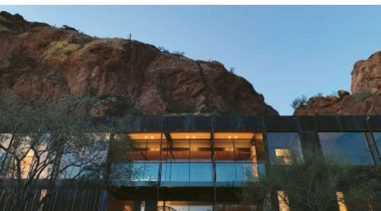
Photo: The Construction Zone
