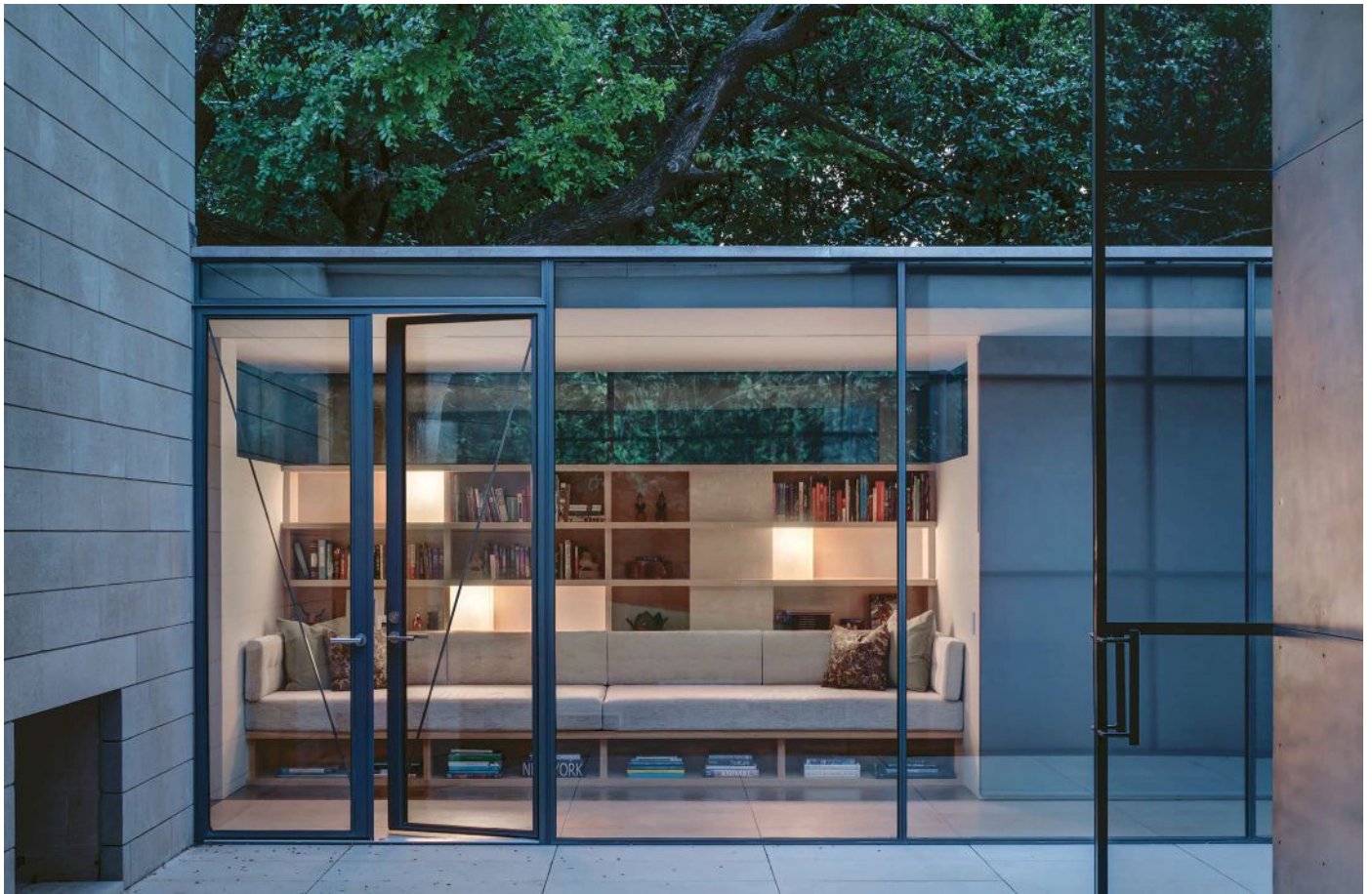
This page: The thin metal roof is cantilevered in an L shape with structural reinforcing on the concrete wall. Frames for the fixed glass were pre-made off-site and the glass bolted in. The units were then hung from the cantilevers on-site to achieve an ultra-slim profile. Staggered bunkbeds strike a sculptural pose as they, too, cantilever.
