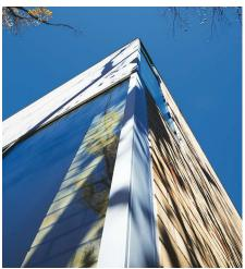
This page: At the back of the house, the garage hides behind cement panels, integrating with rear façade. The interior brick wall terminates a window-frame width from the outside face. The design team devised a custom cap to protect the corner.
