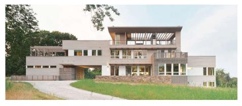
Above: The 2012 Fishers Island House required ferrying modules from the mainland to the island. So, RES4 turned to a system of smaller12-foot-wide modules. The typology used here is a combination double-wide/triple-wide hybrid for a total of 8 boxes and 4,469 square feet.
