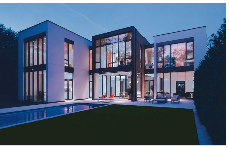
The steel "courtyard" core is flanked by two stucco boxes. A window wall system with roll-up Phantom Screens opens the living room to the backyard oasis for large parties.
