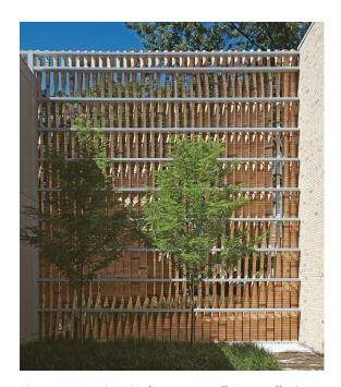
This page: A 4-inch circle of mortar was sufficient to affix the bricks to each other, but wind loads were a concern. Horizontal tubing spaced in 32-inch increments braces the structure. The wall shelters the interior courtyard and private living spaces from view.
