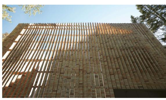
This page: Once a pedestrian material relegated to back alleys, Chicago common brick is celebrated on the façade of this infill courtyard house. Installed in 28-foot columns and rotated at  $\frac{1}{8}$ -,  $\frac{1}{4}$ -, and  $\frac{1}{2}$ -inch turns, the twisted bricks generate a moire effect as people pass by.
