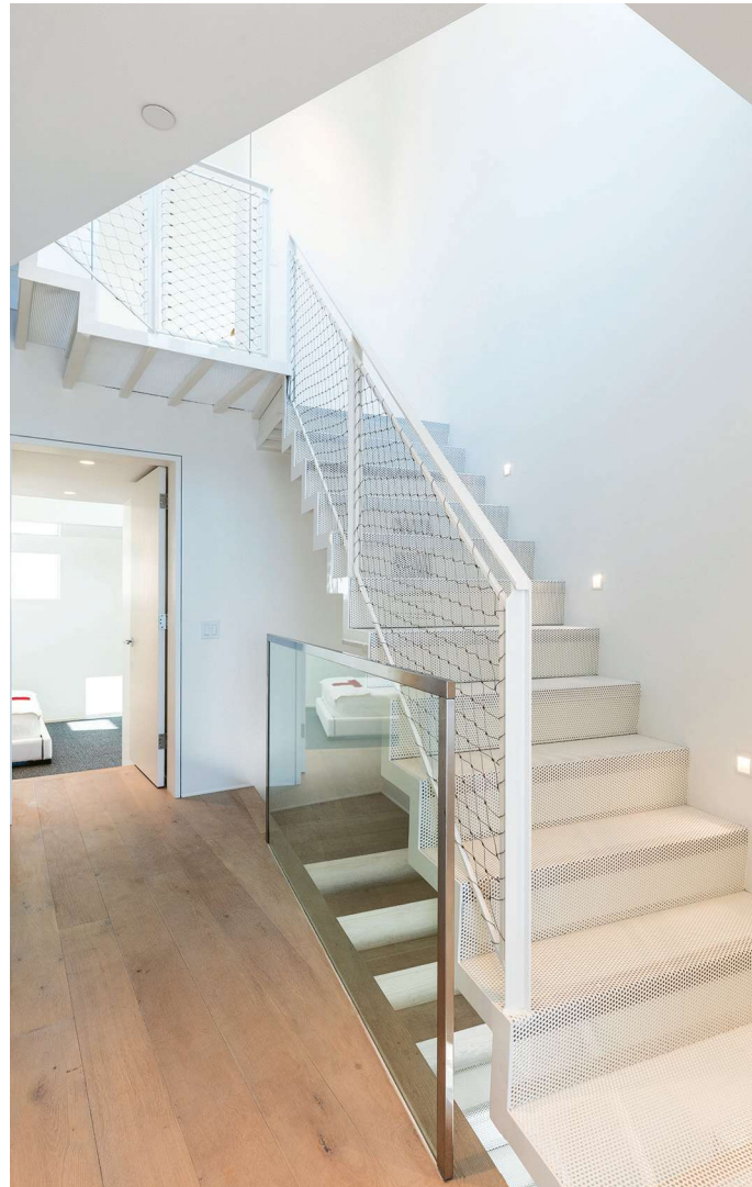
This page: A steel mesh central stair ushers natural light from the roof deck down through the house. When window walls are open on lower levels, it also helps ventilate interiors with fresh sea air.
