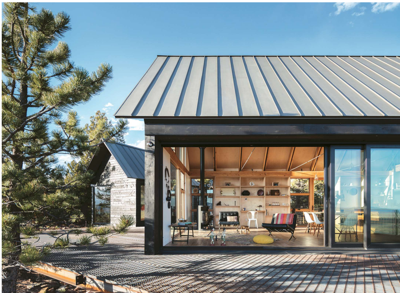
Opposite and this page: To preserve an old pine and grab the best views for key rooms, architect Renée del Gaudio split the three-bedroom plan apart and skewed the two buildings. A metal grating deck links the two volumes, shedding rain and snow.
