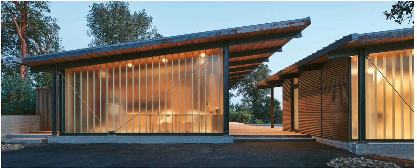
Opposite page and this page: This small, off-the-grid compound occupies only a fraction of its remote 160-acre property outside of Cloverdale, Calif. The clients camped on the land for several years before commissioning a minimalist permanent dwelling.
