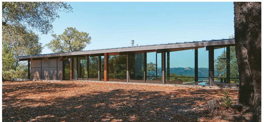
This page: The “pi-shaped” steel beams combine with glazing and channel glass to evoke the lightness and openness of the clients’ former tent life onsite. Metal-clad roofs and fascias guard against wildfire.
