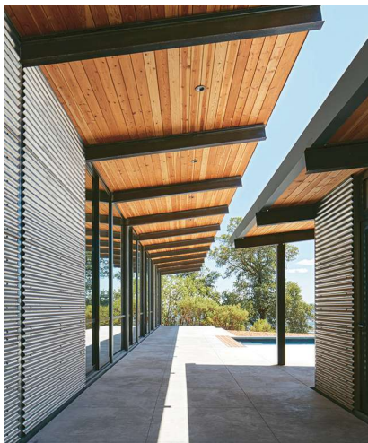
This page: Given the site's remote location and difficult access, a steel structure proved more efficient and practical to build than a wood frame. Deep, almost-touching overhangs protect against rain and sun.
