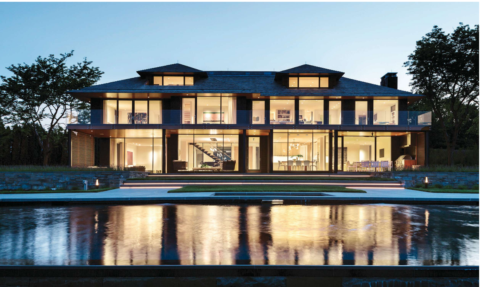
Opposite and this page: The new floor plan showcases manmade art and natural beauty without forcing them into direct competition. Focus on each is carefully orchestrated and facilitated by quiet, skillful architecture.
