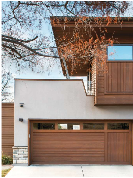
Wedge House is a design-build remodel of a 1973 ranch, resulting in a high-performance house with geothermal heating and photovoltaics.
