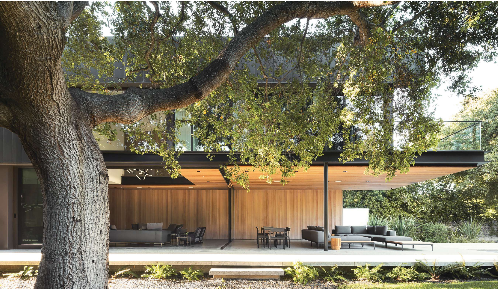
This page: A nearly 4-ton steel beam underpins the living room atrium and supports the master bedroom and deck as they cantilever over the outdoor seating area and into a close-up view of trees and water.
