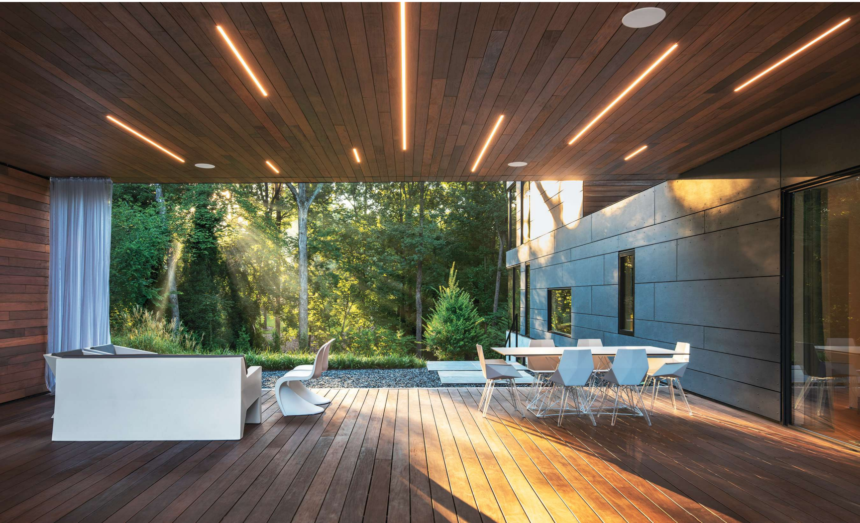
This page: The ipe-lined “hole” created by the split boxes is the home’s tour de force. Breeze travels down the hill from the street, says David, moderating temperatures in the outdoor room.
