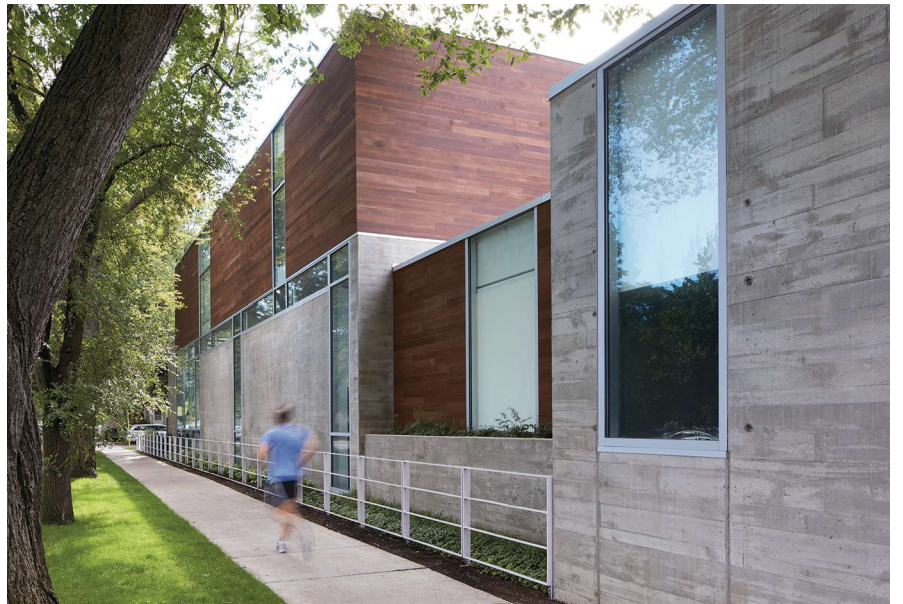
This page and opposite: Not everyone sees the virtues of a corner site, but Mark Peters is a veteran of urban design and the deft balance of competing requirements for daylighting, views, and privacy. From the exterior, public realms appear as sections of board-formed concrete walls and glass; private areas are wrapped in cedar siding punctuated by strategically placed glazing.
