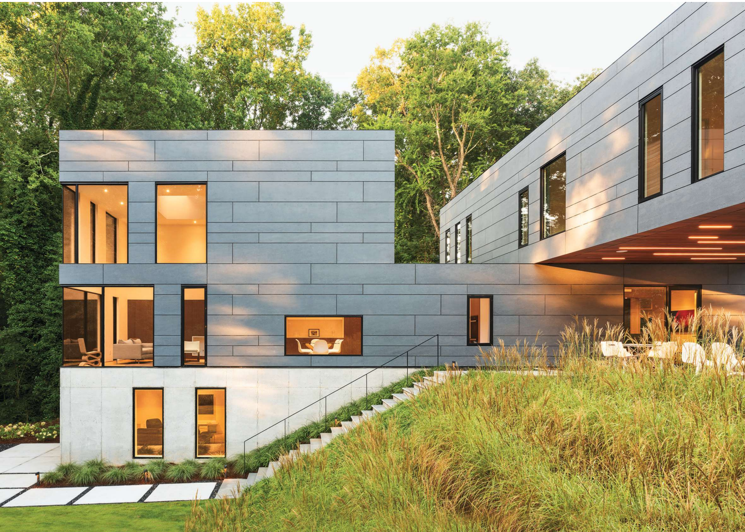
This page: Fiber cement rainscreen cladding, foundation walls, and fenestration arrange in precise patterns to activate the home's otherwise serene exteriors.
