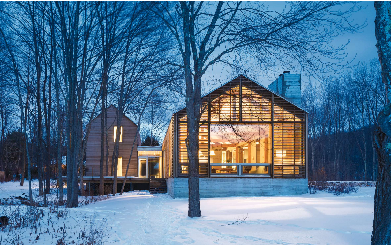
The limited palette of materials is hardy and handsome to withstand harsh winters and active children—board-formed concrete, Western red cedar, and standing seam metal roofing.
