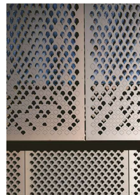
Above: Precast concrete window screens on the original Wallace Neff house inspired the metal library screens.
