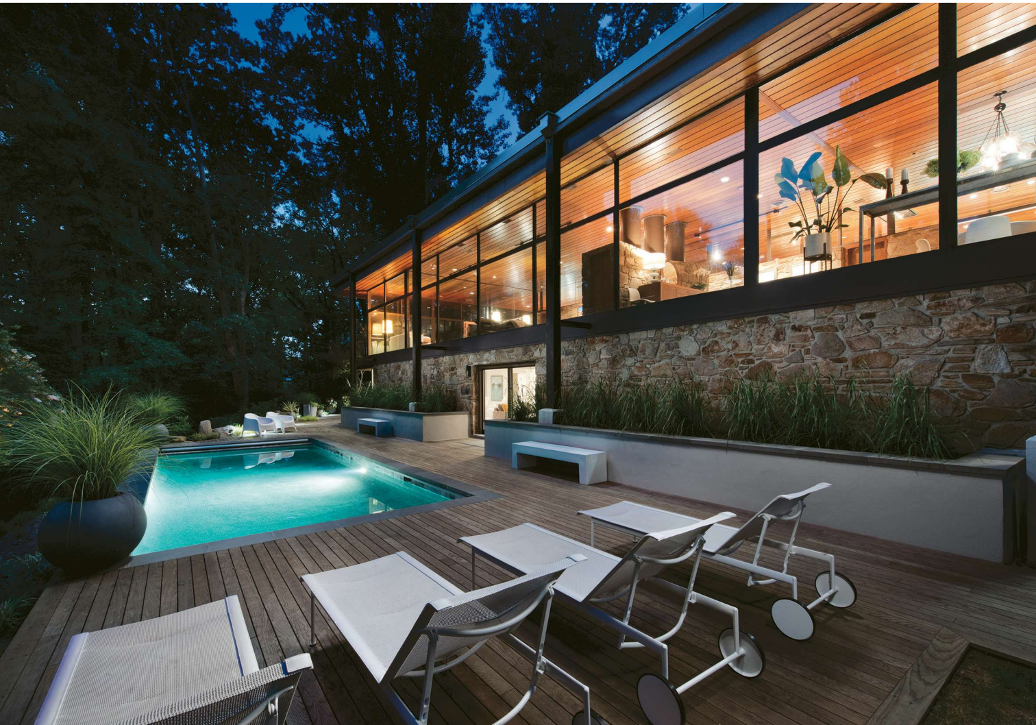
Above: Rethinking and expanding the outdoor landscaped areas was a chief goal of the renovation. New sliding doors connect the lower level to a new pool and terrace. Beyond the cultivated outdoor areas, the woods reclaim the land.
