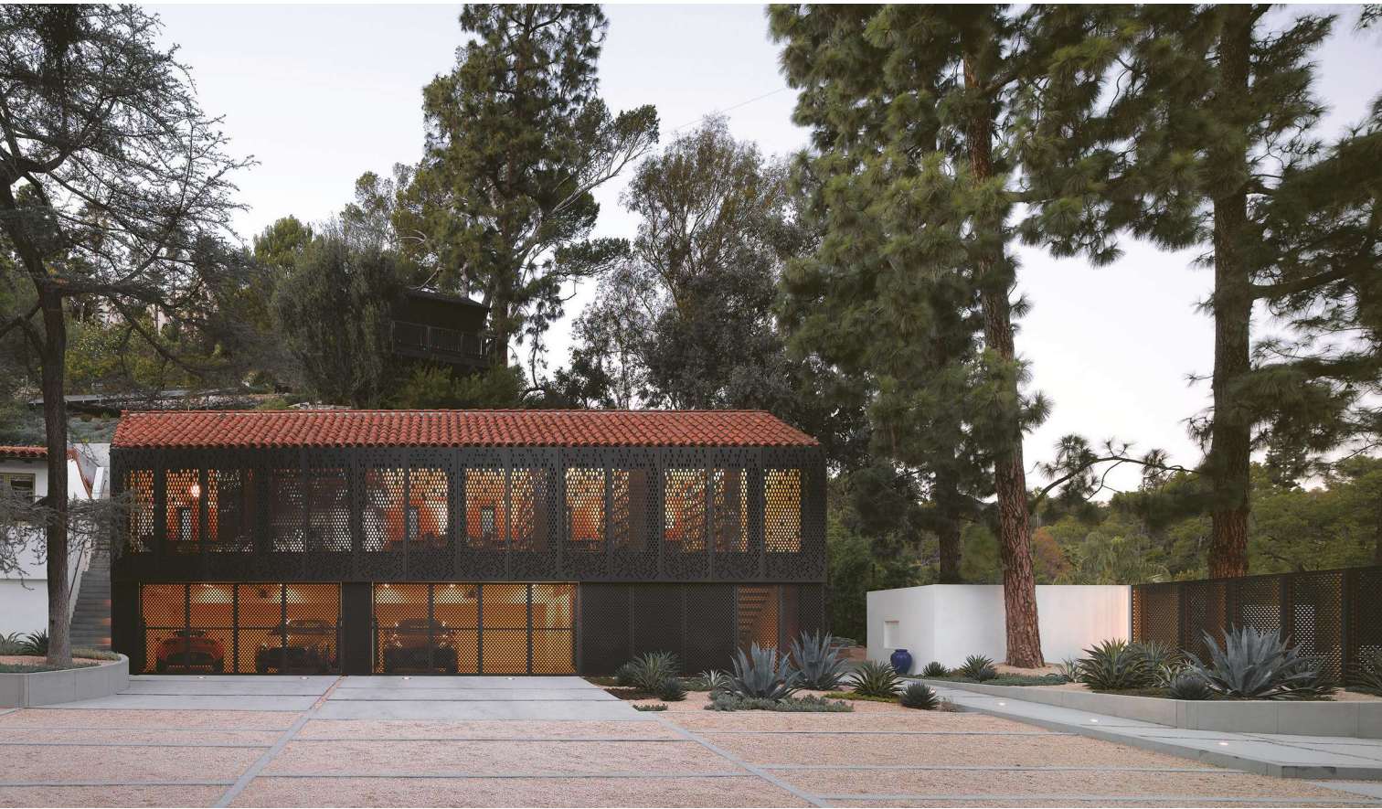
The screen façade appears almost solid by day, but shimmers at night, exuding warm and welcoming light.
