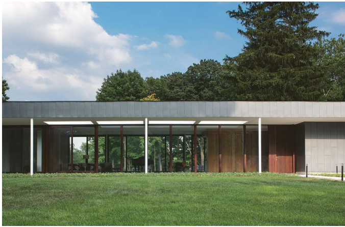
This page: The house is a tightly orchestrated study in transparency. Deep overhangs control glare inside.
