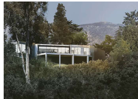
Project: Las Alturas Residence; architect: Patrick Tighe, FAIA, Tighe Architecture, Los Angeles. Drawings: Tighe Architecture
