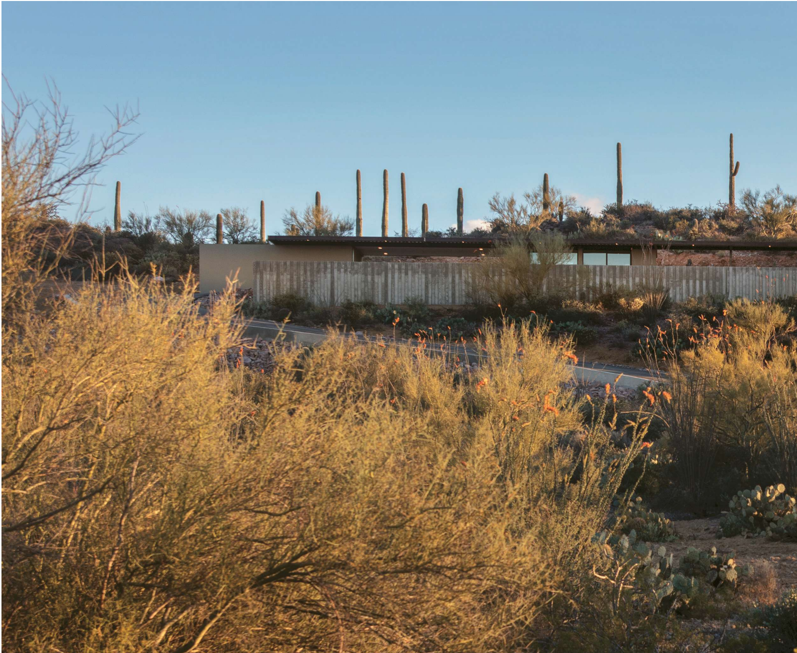
Above and right: Steeped in the lessons of Taliesin and Frank Lloyd Wright, the architects designed a house of the hill and not on the hill. A 17-foot cantilever focuses the living room on the panoramic desert view.
