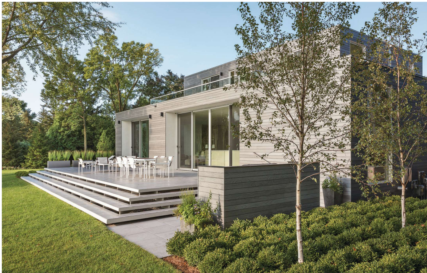
Above: The architects chose weathered Accoya wood siding, which was "burnt, brushed, and stained." Viewed close up, it mimics the lively shimmer of lake waters.
