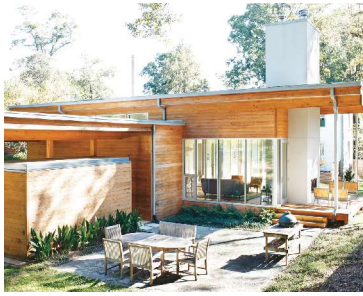
Above: Lightroom pursues sustainable strategies that rely only lightly on the grid.
