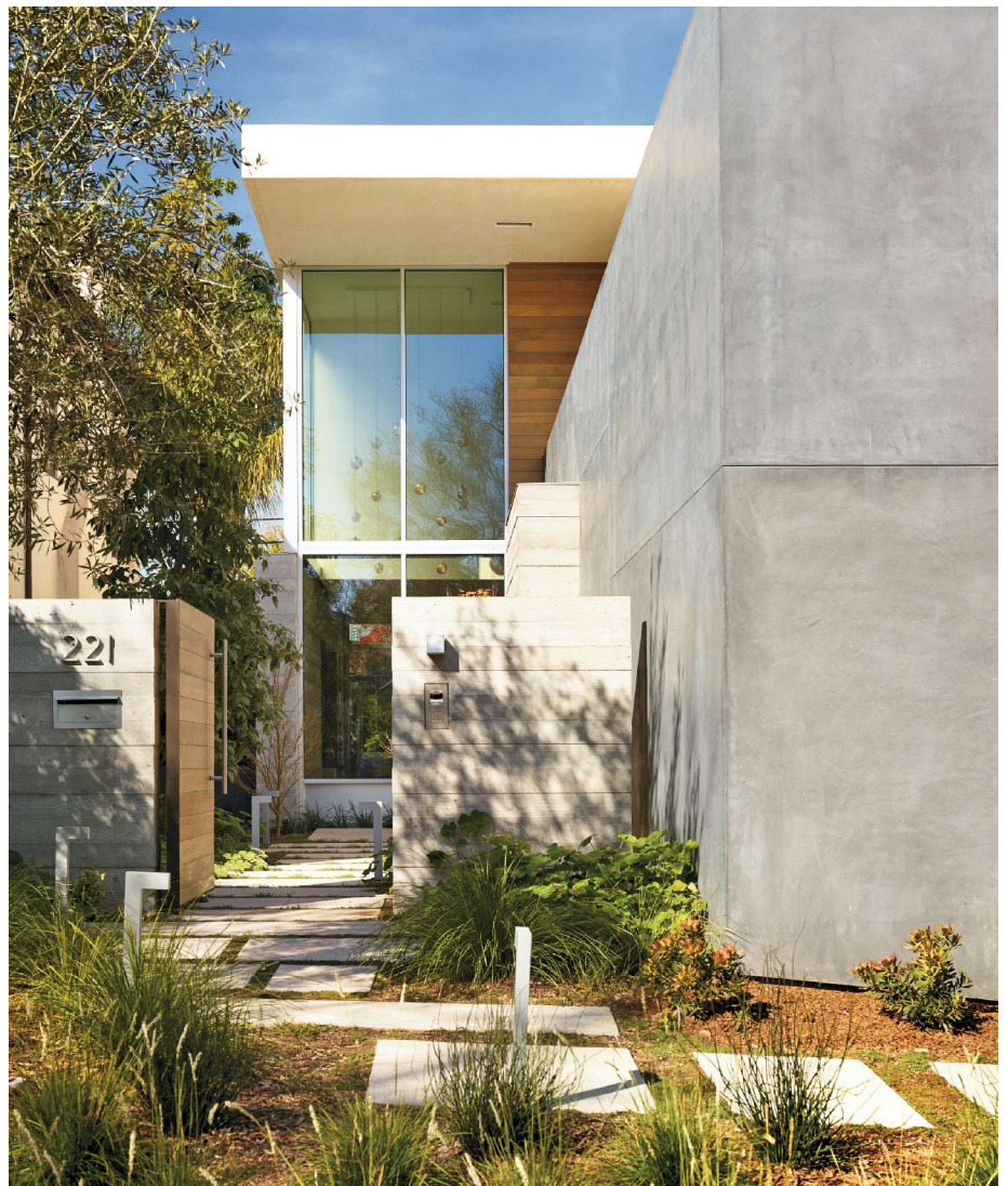
Above: The front entry is pulled back from the street and into a small courtyard, creating a peaceful procession from public to private space.
