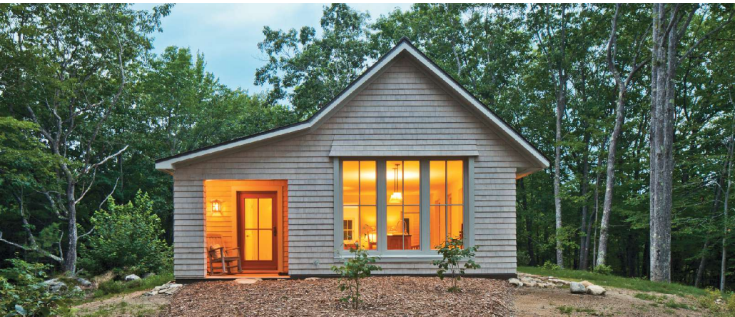
Above and right: GO Logic's custom work inspired many houses in its prefab portfolio. House on a Knoll is a 1,000-square-foot, single-level plan with two bedrooms, a bath, and a screened porch. Below right: The secret sauce for the company's thick, passive house walls and super-insulated foundations.
