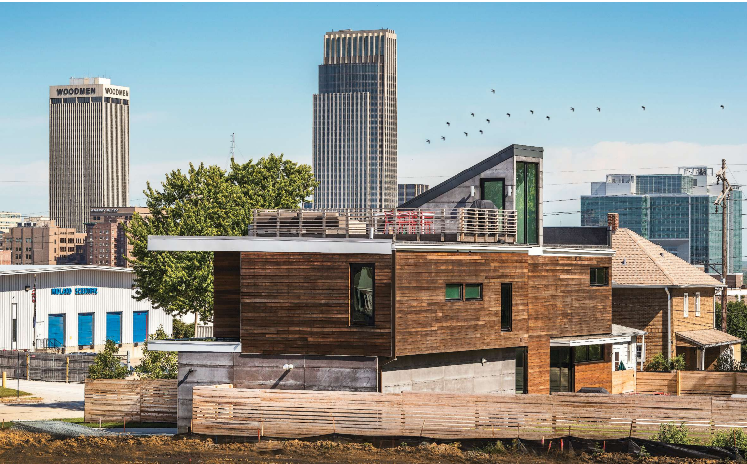
Above: The architects tested the roof monitor with a crane to locate it optimally for windows and views. The roof deck has sweeping skyline views of Omaha.
