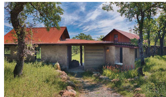
Above: Arkin Tilt's plaster supplier noted that the pink hue on the walls is from the fire heat drawing out the natural iron oxides. The soot brushes off.
