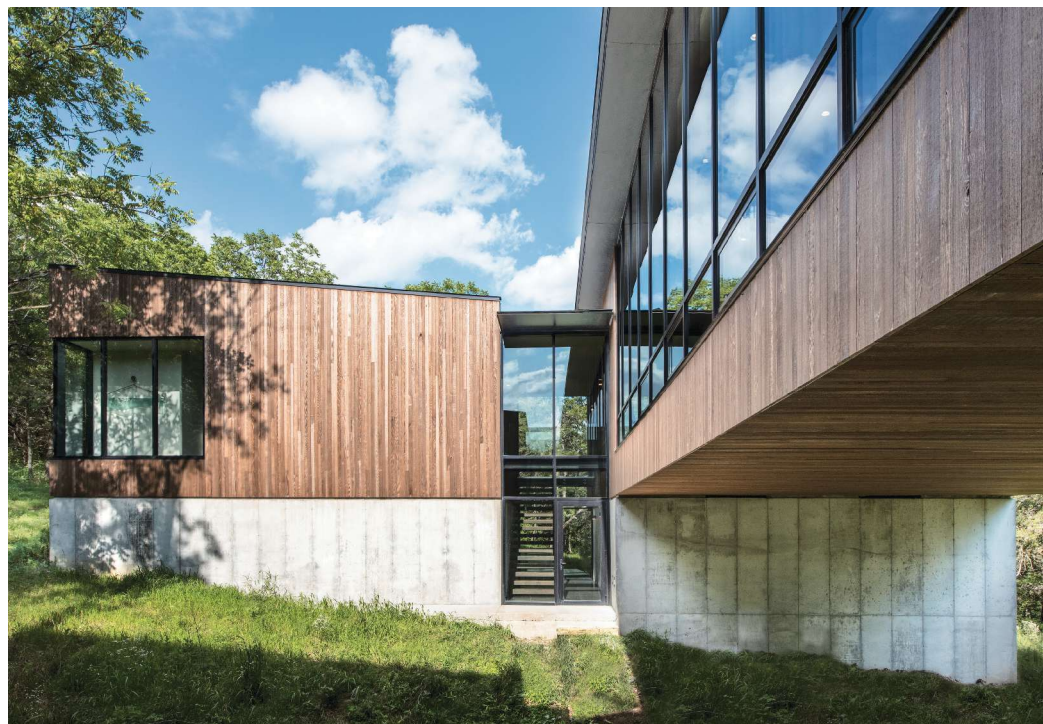
Above: Stairs off the bridge lead to a lower level where family space will be built out later. A tall concrete plinth keeps more vulnerable materials up above the snow line.
