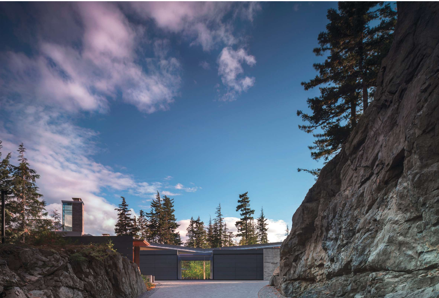
Above and below: Between a wedge of rocky ledges is the motor court and entry to the insular property. The low-slung clad buildings are actually garages. At their center, an opening topped in blue architectural glass leads to the front lawn and the home's big reveal.
