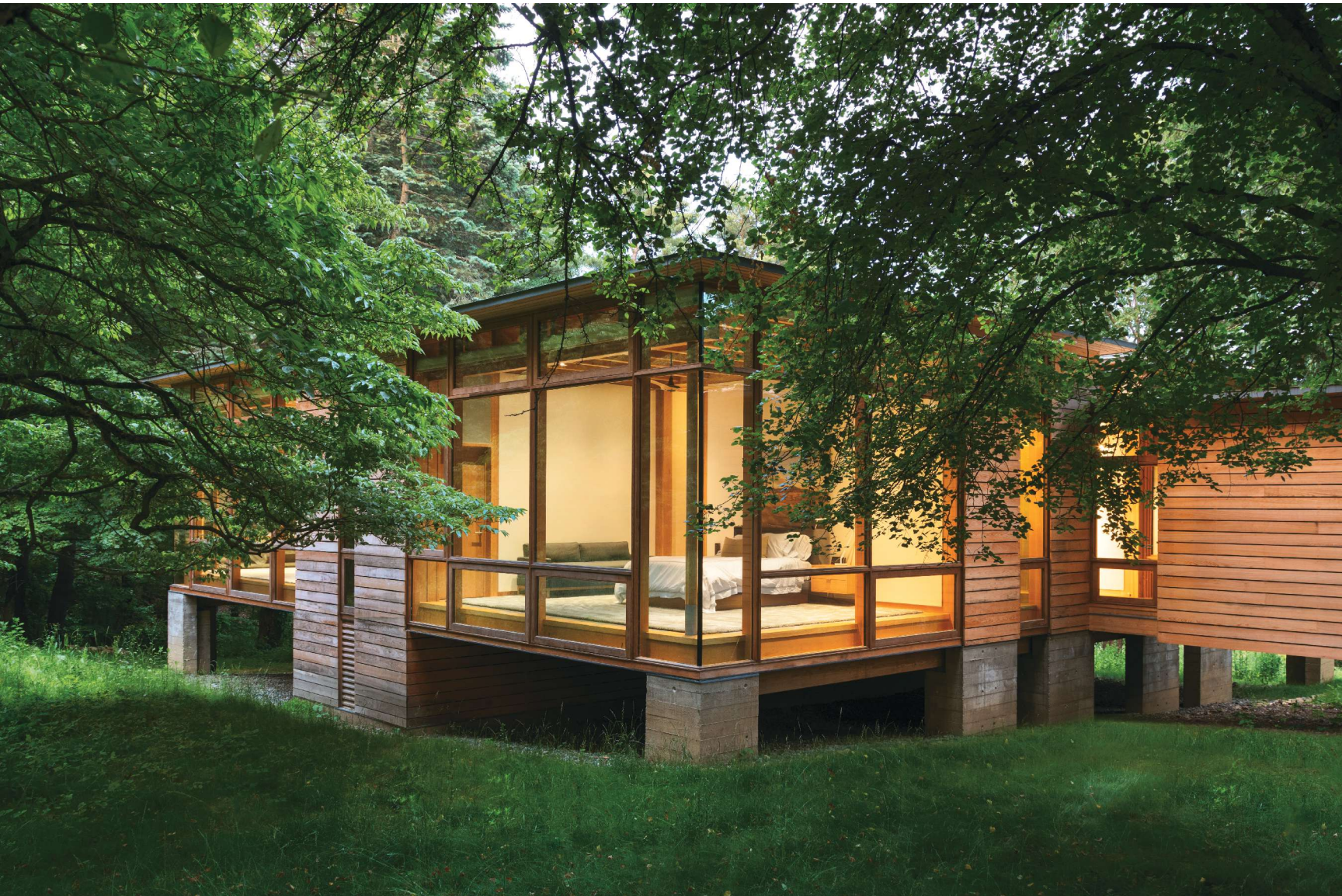
Clockwise from above: Architect Jim Cutler elevated the house on concrete piers so it could navigate the contours of the site without level changes.
