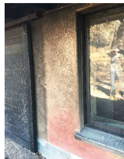
Above: Arkin Tilt's plaster supplier noted that the pink hue on the walls is from the fire heat drawing out the natural iron oxides. The soot brushes off.
