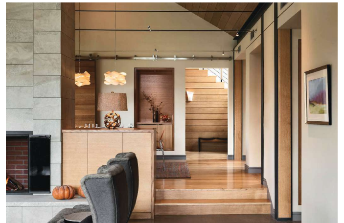
Clockwise from opposite page: Steel columns and beams, wood ceiling panels, and polished concrete floors extend from the covered porch inside to the living room. In the living area, the steel columns are inset with wood. Two steps up from the living room, the dining area marks a flooring change to wood. The wood floors continue up the stair wall of the family wing.
