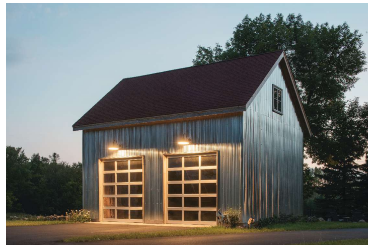
Above: Existing buildings were refurbished, repurposed, or reconstructed. Material from an existing grainery was salvaged for the new garage.
