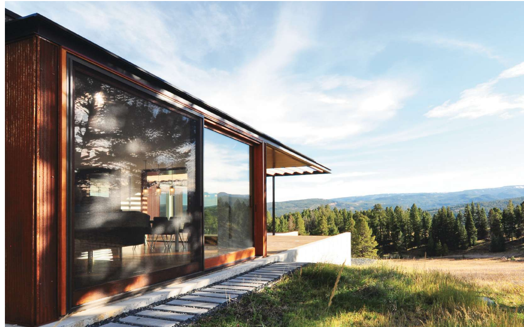
Above: Looking out on the Rocky Mountains in the distance, Mountain House embraces the changes its corrugated Cor-Ten steel exterior will undergo as it ages.
