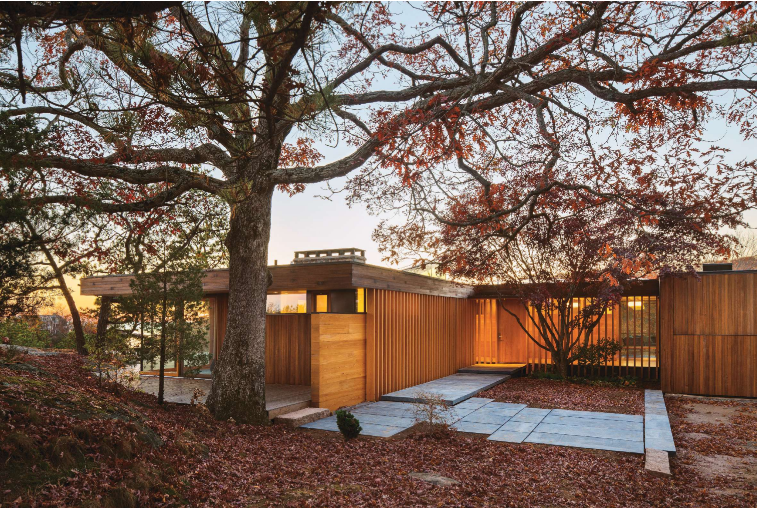
Above: Cypress boards laminated in triple thickness delay the full reveal of the interiors. Visitors can see straight in but not at an angle.
