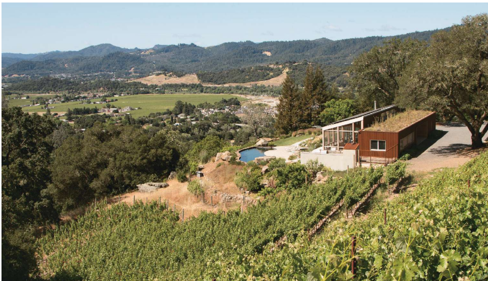
Opposite: Wrapped in COR-TEN steel, the front entry is quietly welcoming—and handicapped accessible. Top: The great room segues into the screened porch, which provides protected access to the guest bedrooms. Above: Occupying the footprint of the original log house, the new Cloverdale Residence has panoramic views of northern Sonoma wine country.
