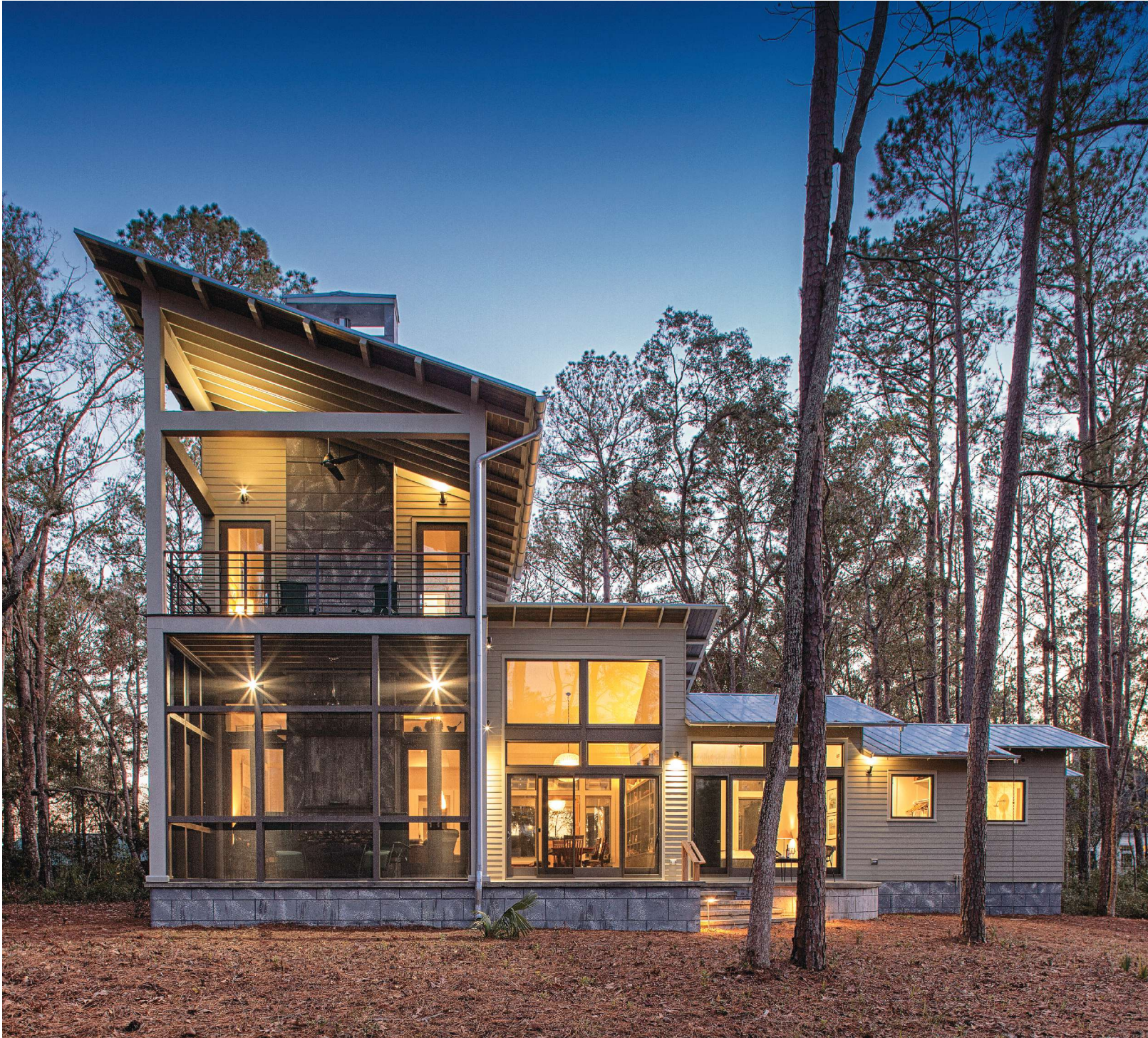
Above: Set back 60 feet from tidal waters, T House captures long views north across Dataw Island's marshy low country to the water. Deep roof overhangs help protect the house from frequent summer storms.
