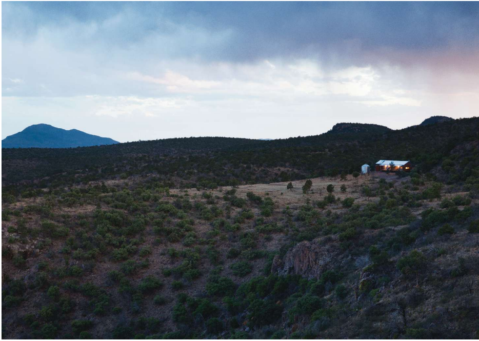
Above: Located in remote Marfa, Texas, the recent Prow Porch House was site assembled and built off the grid with fire-resistant materials.
