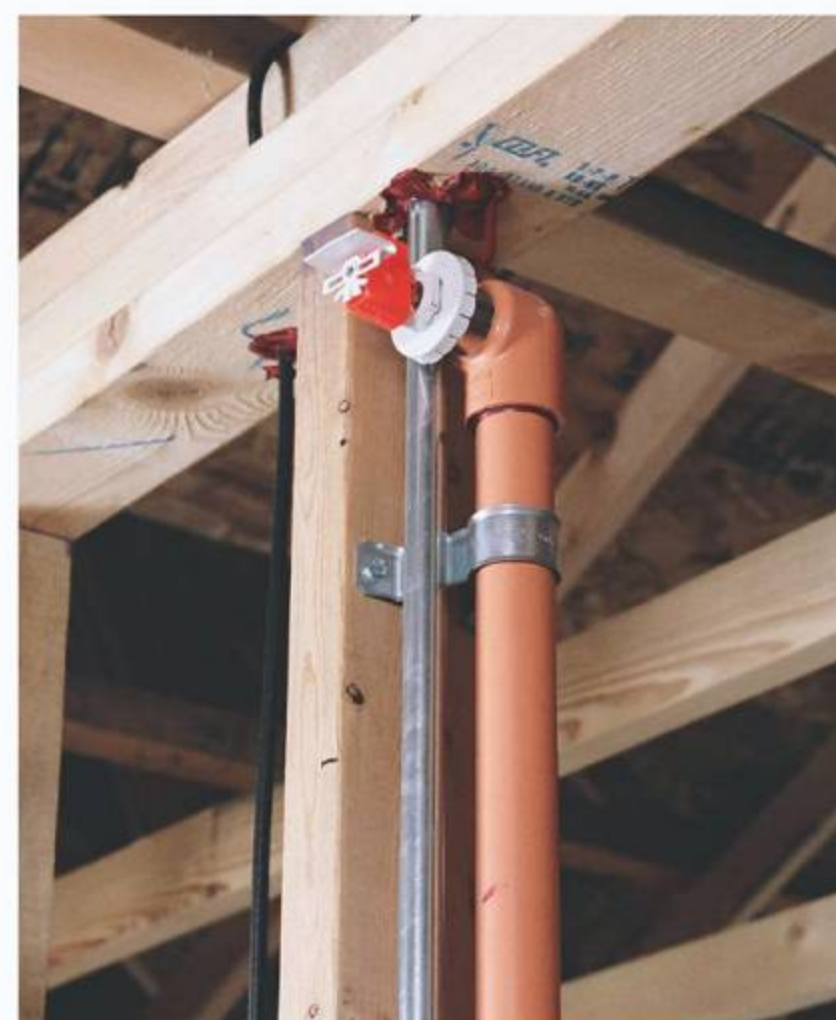
↑ One of two installation options, stand-alone fire sprinkler systems are connected separately to incoming water supply and operate independently from domestic water lines.
