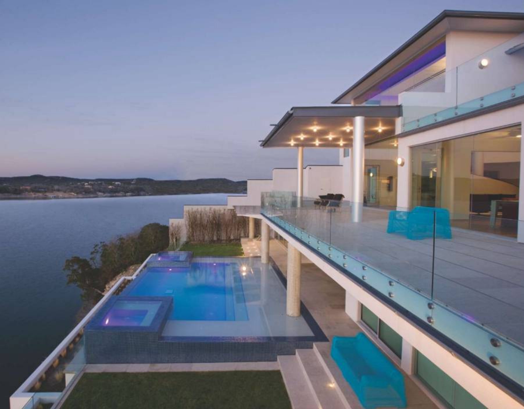
The cutout pattern from the front window panels is seen above the back patio (inset left). The wind coming off this Texas lake can be fierce, which required custom anchoring systems to be created.
