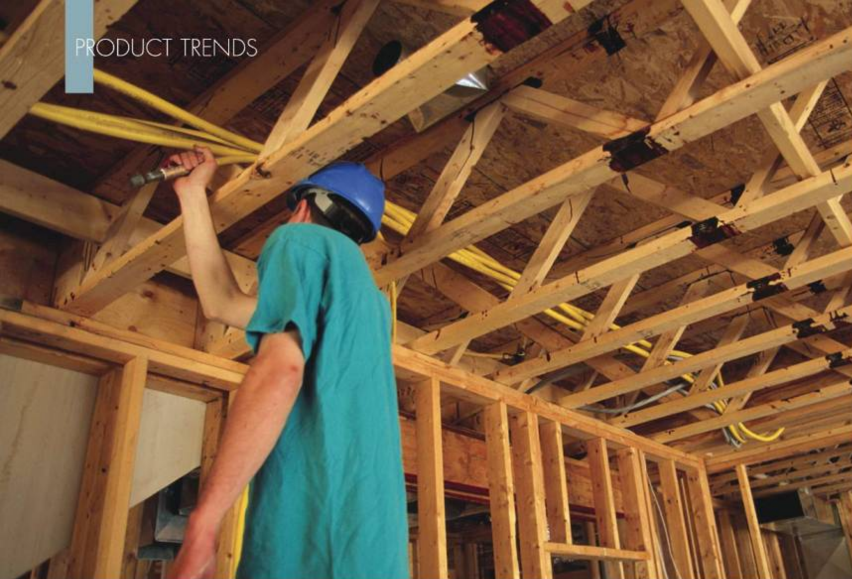
The Open Joist truss from Universal Forest Products is an all-wood, finger-jointed, non-plated truss with space to slide wire, ductwork, pipe or other mechanical components.
