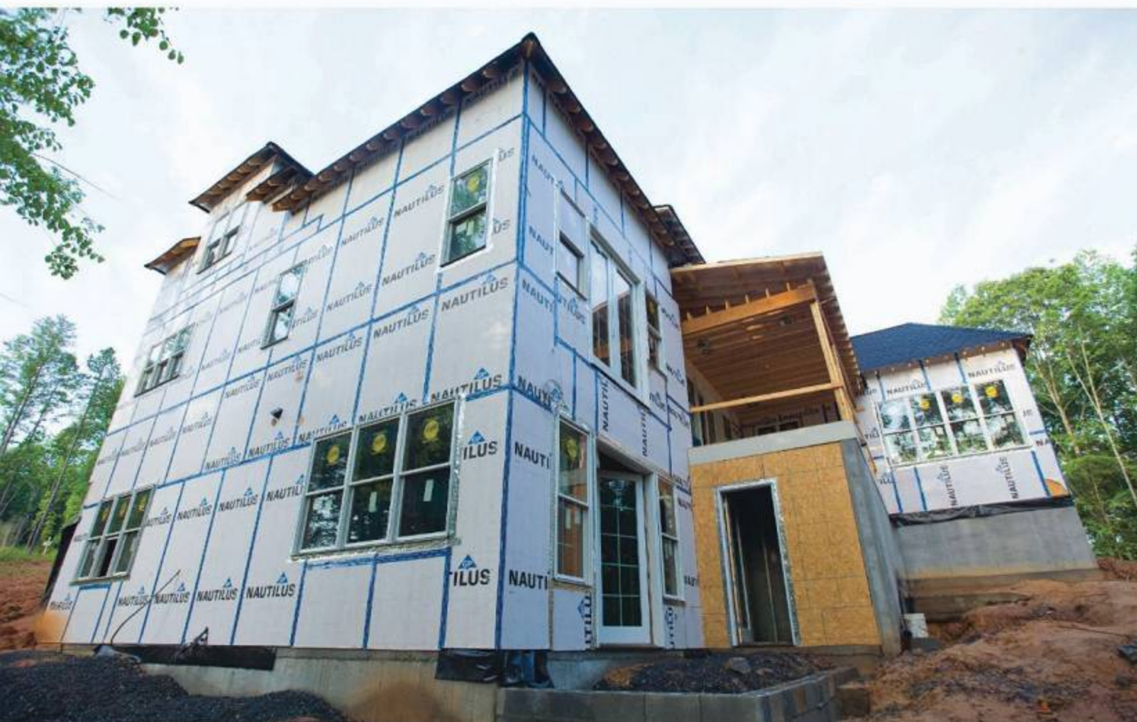
Nautilus sheathing by Georgia-Pacific comes with preapplied weather barrier that can be peeled back and reapplied, which is convenient for finishing window openings.
