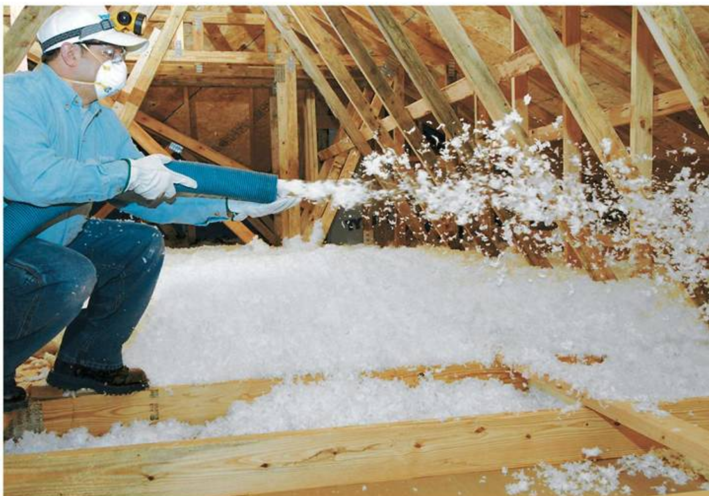
CertainTeed's InsulSafe SP is a fiberglass blowing insulation used in residential and commercial construction as a thermal and sound-absorbing insulation. It is designed for pneumatic installation in open (attic) and closed (sidewalls/floor) construction cavities.
