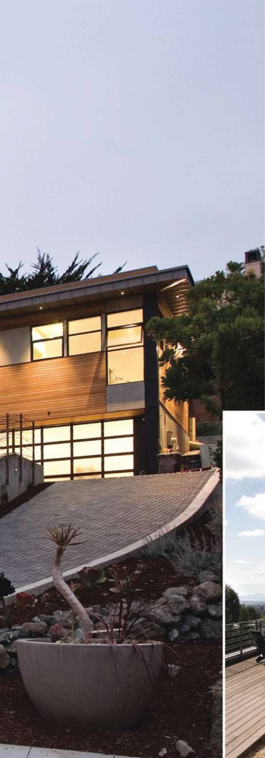
The Margarido House, as it's known, is the only LEED Platinum home north of Monterey, Calif. It's also GreenPoint certified by BuildItGreen.org. A NanaWall folding door (seen in inset) expands living space to the backyard where access to the rooftop garden is gained via an outside staircase.
