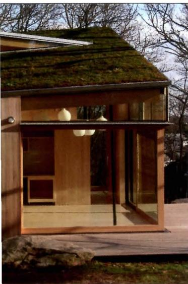
On approach, the sod roof tips up, preserving the building's scale while allowing for head clearances upstairs. Transparent eaves help the cottage blend with the landscape.
