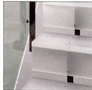
The view from the lower level up through the top-floor skylight shows how the staircase distributes light throughout the house. One-inch gaps beneath each riser (left) enhance the effect of airiness and transparency.
