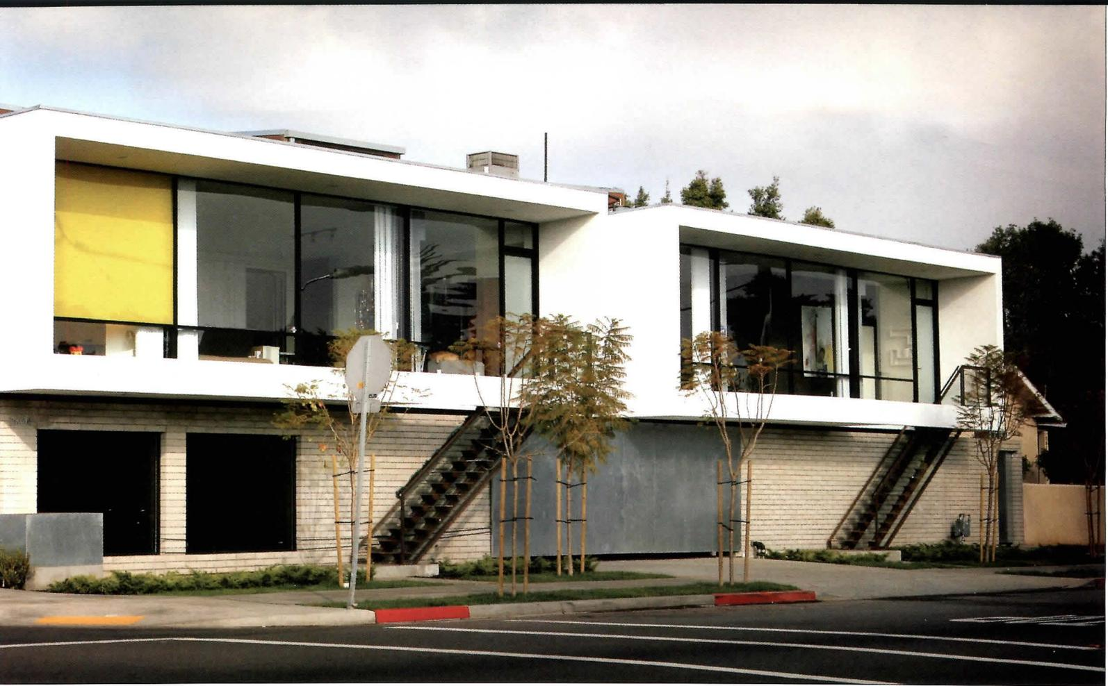
A welcome newcomer to the neighborhood, K Lofts adapts a derelict commercial structure and reuses it for market-rate and very low-income housing. Built for less than \$100 per square foot, the project uses materials—concrete, stucco, and mild steel that resembles Corten—in innovative ways.
