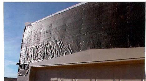
The wrinkles in the Secondary Weatherproof Membrane will cause thick and thin spots in the basecoat. These will have different expansion and contraction characteristics side by side and will stress the stucco assembly.
