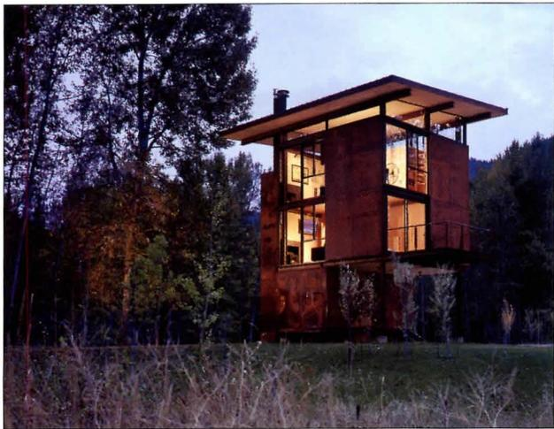
Flood-proof and virtually indestructible, this steel-and-concrete cabin perches on the floodplain of a 43-acre site. It's shielded with huge steel shutters that can be closed with a handwheel when the owners leave (top left).
