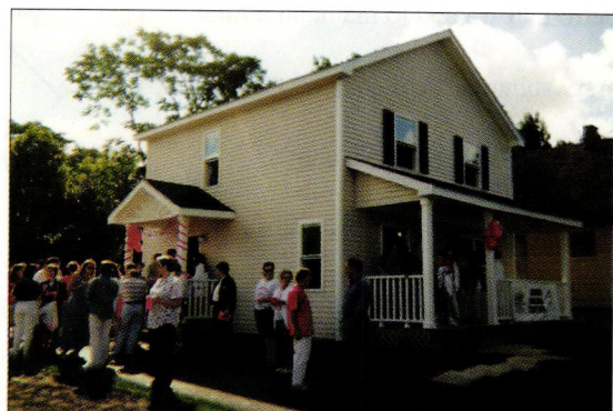
Courtesy Greater Living Architecture Habitat for Humanity built this house in Rochester, N.Y., from plans donated by Greater Living Architecture.
