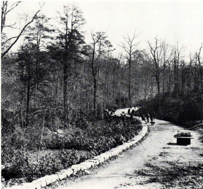
3. A portion of the approach road under construction in about 1892.
