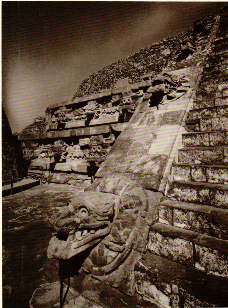
4. Teotihuacán, stepped platform of cantilevered panels on talus bases.
