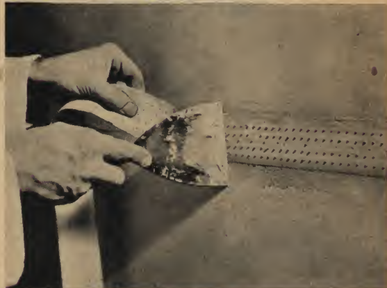
Perforated PERF-A-TAPE is pressed into the cement
