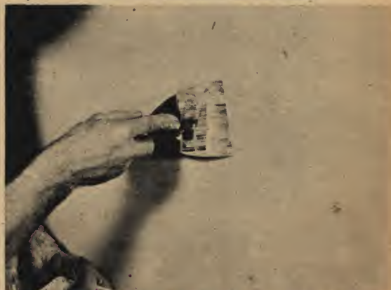
Finishing coats of cement are applied and feather-edged
