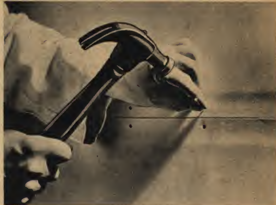
Note recessed channel in which SHEETROCK is being nailed
