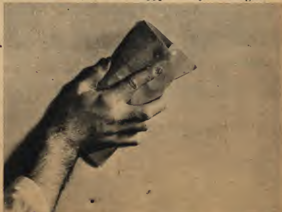
After drying the joint is sanded smooth
