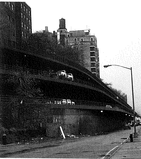
Traffic on the Brooklyn-Queens Expressway ducks onto two decks cantilevered from a cliff and covered by the Brooklyn Heights Promenade. When engineers proposed the freeway structure, Moses added the promenade.
