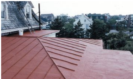
This metal roof has been treated with a waterproofing, elastomeric Acrymax coating from Preservation Products .
