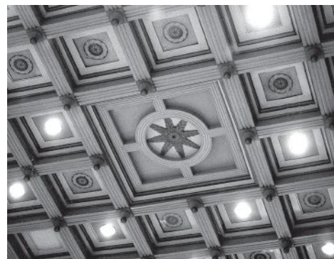
NIKO fabricated and installed these pressed-metal coffers.
