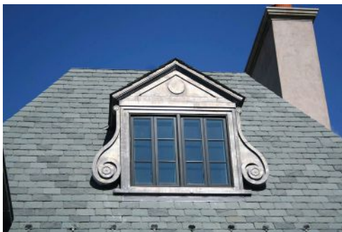
This dormer was created by Slate and Copper Services .
