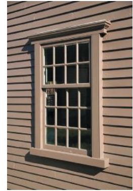
Architectural Components restored the windows for the Jacob Whittemore House at the Minuteman National Historic Park in Lexington, MA.
