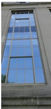
Pilkington NA's vacuum insulated glass was used as part of a restoration project.
