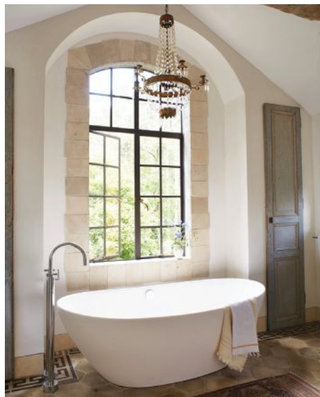
Seekircher Steel Window restored the French casement windows and brass hardware in this private home, left. Below, A Manhattan penthouse features a row of single and double casements flanked by vintage doors. Seekircher Steel Window restored them.
