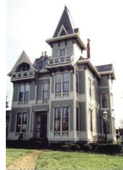
The Dankenbring residence in Cincinnati, Ohio, features Historic-One-Lite HOL-B storm windows in a custom color by Allied Window .
