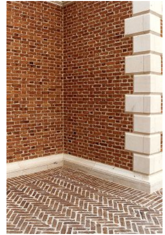
Old Carolina Brick Co. supplies handmade, coal-fired brick that can be used for both paving and wall facing.
