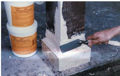
WoodEpox from Abatron can be used to repair wood elements.
