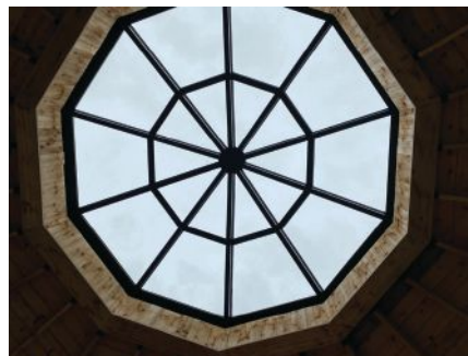
Glass House constructed this circular skylight.
