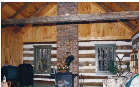
This 45 x 34-ft. barn was constructed by Sylvan Brandt using four bents and eight major outside posts, most of which are hand-hewn hardwood.
