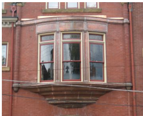
NIKO Contracting Co., Inc. fabricated and installed this custom copper radiused bay window surround.
