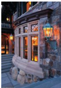
Hope's Windows were specified for the five fixed curved-on-plan windows which are located near the first-floor entry and provide sweeping views of the lake. They were curved to a modest inside radius of 201-3/8" and were glazed with curved-on-plan glass to fit frames measuring 22 by 61.
