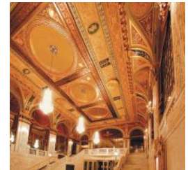
Conrad Schmitt Studios' restoration work at the previously abandoned Palace Theatre (Thomas Lamb, 1922) in Waterbury, CT, included ornamental plaster and scagliola, decorative painting, millwork and metal work.
