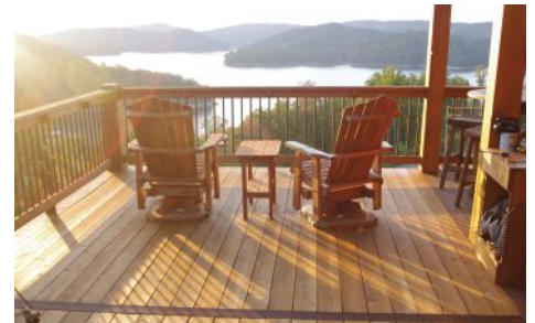
This house is all timber frame. It has 1 x 4 porch flooring, 5/4 x 6 decking and 1 x 8 bevel siding, all AB grade Siberian Larch provided by Stein Wood Products .
