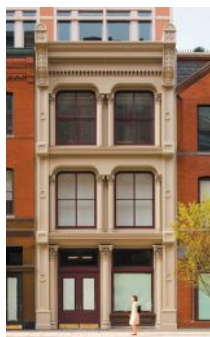
Robinson Iron cast and fabricated this new storefront façade in aluminum to match the surrounding historic neighborhood in Washington, DC.
