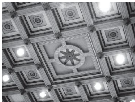
NIKO fabricated and installed these pressed-metal coffers.
