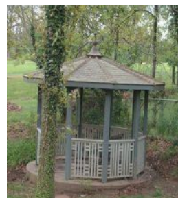
This gazebo features W.F. Norman's Style "A" shingles with its continuous hip finish and a custom-made finial on top.
