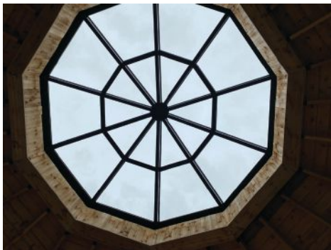
Glass House constructed this circular skylight
