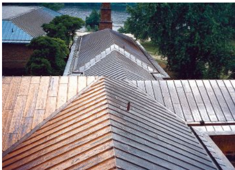
NIKO Contracting Co., Inc. installed this batten-seam and flat-lock copper roof.
