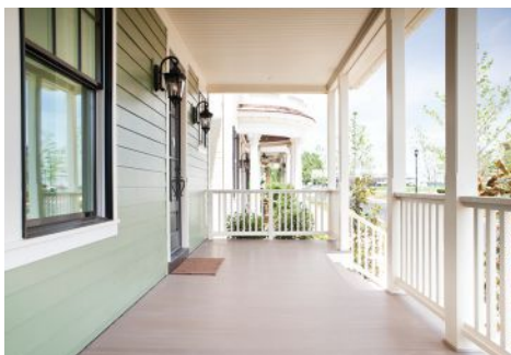
Aeratis solid PVC tongue-and-groove porch flooring was chosen for this home due to its durability and ability to hold paint colors and still maintain its warranty—and it is the only product that maintains its warranty when installed in a waterproof application.
