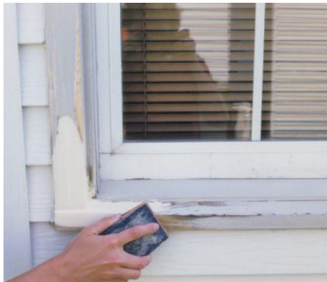
Abatron's LiquidWood restoration system regenerates and waterproofs dried out or spongy wood.
