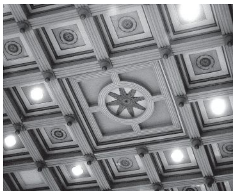
NIKO fabricated and installed these pressed-metal coffers.
