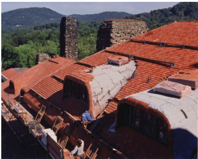
Craftspeople installed the Ludowici multi-hued red clay tile for this roof in Asheville, NC.
