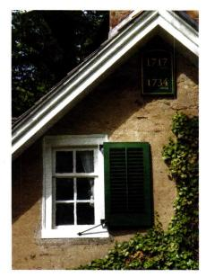
Timberlane handcrafted this traditional louvered shutter; it is adorned with a tilt-rod and period-accurate . hardware.
