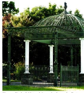
Wiemann Metalcraft fabricated this gazebo, fence and trellis in cast and wrought iron.
