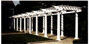
This pergola from Chadsworth was fabricated from cellular-PVC beams and rafters and PolyStone support columns.
