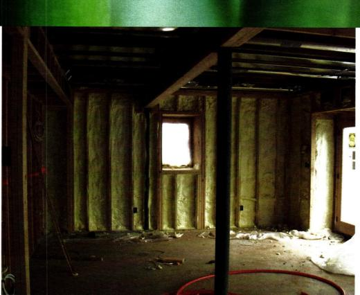
Closed-cell insulation is sprayed onto the exterior masonry wall in a recent barn conversion project by VMA.
