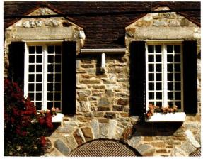
Shuttercraft's mortise-and-tenon shutters can be mounted on stone, as shown here, and are available with moveable and fixed louvers.
