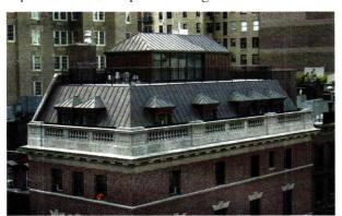
NIKO fabricated the copper dormers and mansard roof and also installed the copper penthouse for this building in New York City.
