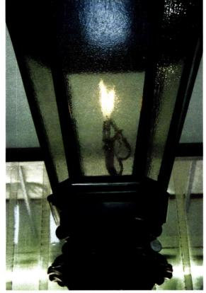
Historical Arts & Casting custom fabricated this cast-metal gasburning lantern.
