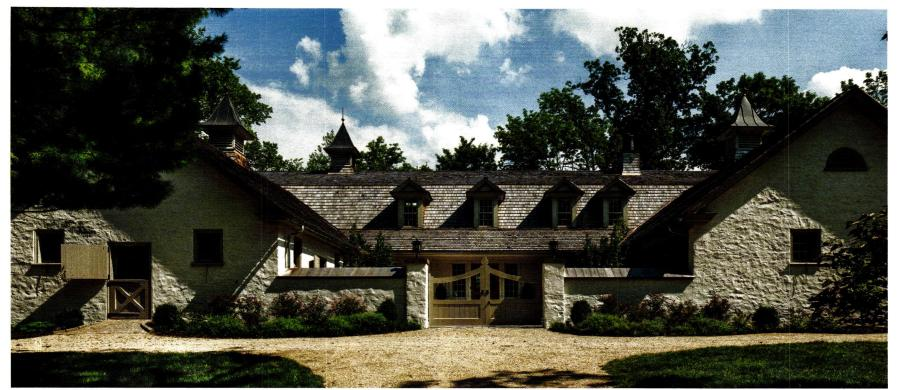
The stucco exterior was cleaned and repaired and is complemented with new jumbo taper-sawn cedar shingles and pointed cupola caps, the latter of which are common to racing stables.
