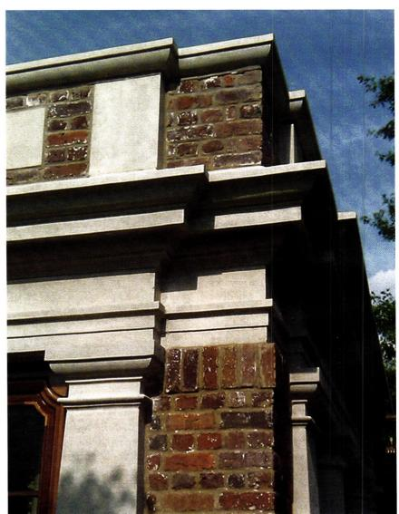
Internal downspouts at the corners of the folly wash the water to the ground, giving the illusion that the single-room building is a thing of the distant past.
