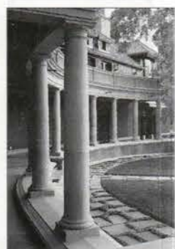
Columns and capitals in GFRG, manufactured by ARCHITECTURAL FACADES UNLIMITED, are featured in this curved colonnade. Write in No. 1470
