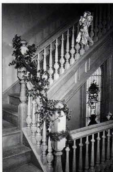
Made of quarter-sawn white oak, this Victorian reproduction staircase was created by ARCHITECTURAL STAIRBUILDING.
