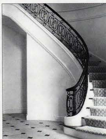
SCHWARTZ'S FORGE & METALWORKS fabricated this ornate stair railing with a mahogany cap for a residence in Greenwich, Conn. Write in No. 1218
