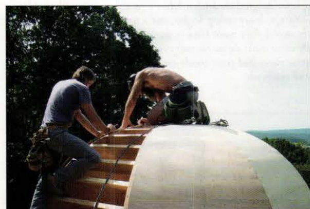
Installing the copper roof on the octagonal tower was a difficult job, not only because of the 50-ft. height of the tower, but also because of its eight-sided shape. It was installed by Mark Sauer Contracting of Caldwell, N.J.
