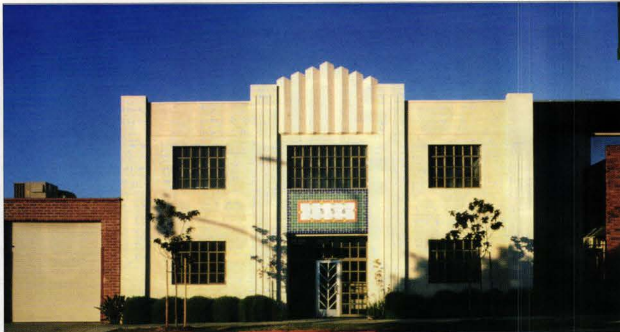
Further proof of the versatility of Appleton & Associates: Marc modeled the firm's own office building to resemble an adaptively reused, Art Deco commercial structure. (Photo: Alex Vertikoff)
