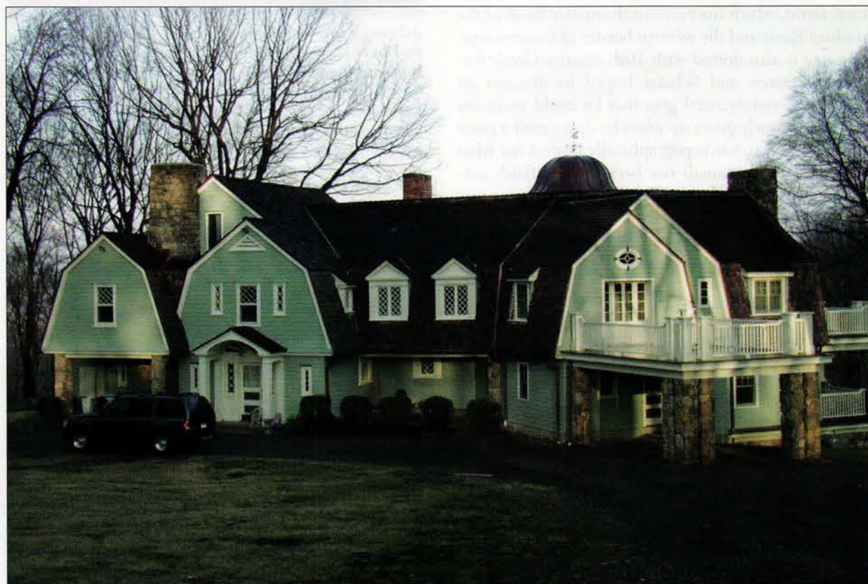
The original gambrel roof line was repeated to maintain the style of the house, as shown in this view of the front entrance, with the addition to the right. The porte cochere features a balcony above and to the far right, the family-room and master-bedroom balconies are visible. The copper roof and weathervane on the tower are also visible over the roof.
