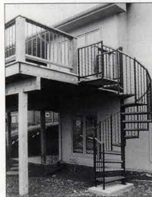
GODDARD MANUFACTURING created this custom-designed exterior spiral metal staircase to provide access to the second-floor balcony. Write in No. 4780
