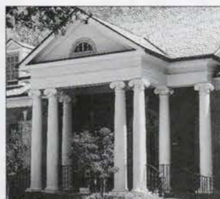
CHADSWORTH'S 1.800.COLUMNNS created these 16-in.-x-12-ft. plain tapered-shaft columns with Greek Erechtheum capitals and Doric bases to grace the entrance of this home in Wilmington, N.C. Write in No. 1580
