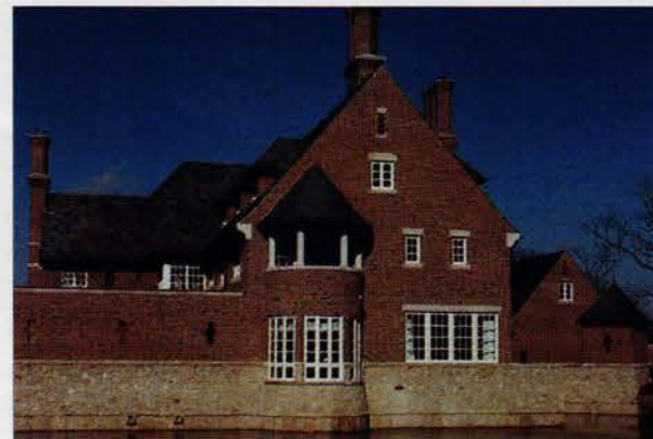
The textured slate roof on this Cotswold-style mansion in Ohio was installed by the DURABLE SLATE CO. Write in No. 3720
