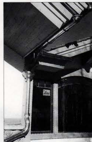
PARK CITY RAIN GUTTER was able to solve this particular drainage situation with these Minoletti copper rain gutters and accessories which are imported from Italy. Write in No. 832
