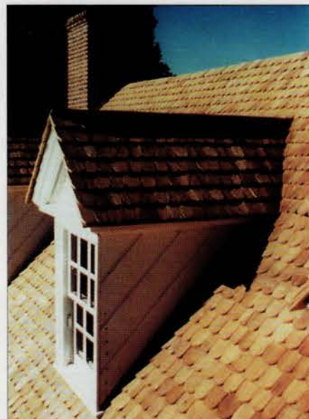
These heart-cypress shingles were fabricated by BARBER LUMBER and installed at Mt. Vernon, George Washington's estate. Write in No. 8074
