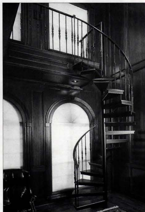
This beautiful spiral staircase made by STAIRWAYS features the company's model #60S oval mahogany handrail, model #326 3/4-in. steel balusters, and mahogany treads. Write in No. 4870
