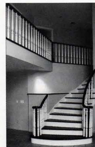
L.P. STAIRS & RAILS fabricated this wood staircase using dark-stained cherry treads, handrail and newel posts, with poplar risers and balusters.
