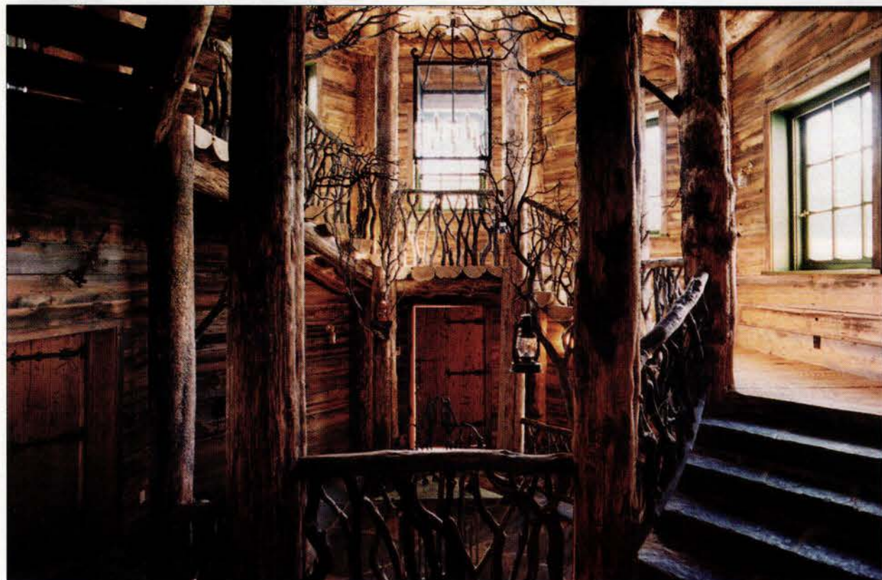
A fantastical exercise in wood recycling, for a real-estate executive's Colorado vacation retreat: The house is clad in salvaged barn siding and supported by hand-been antique timbers; the staircase's columns are Montana standing-dead pine trunks, the balusters are twigs, the treads are split logs, and lanterns hang from branches of California trees damaged in fires. (Photo: Alex Vertikoff)
