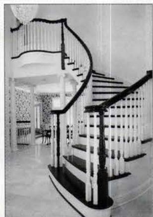
Created by ACORN STAIR & WOODWORK for a residence in St. Louis, this elegant staircase features cherry bandrails, treads and newel posts; the painted parts are made of poplar.
