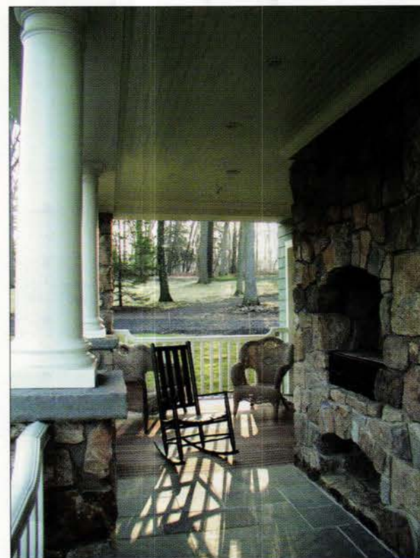
The double-hearth fireplace opens both onto the porch, shown here, and onto the family room. The chimney and foundation are crafted of Modified Bernardsville, a local brown fieldstone supplied by Gladstone Masonry and Stonework, Gladstone, N.J. The masonry work was done by Mar-Mac-Mar, Inc., Newark, N.J.
