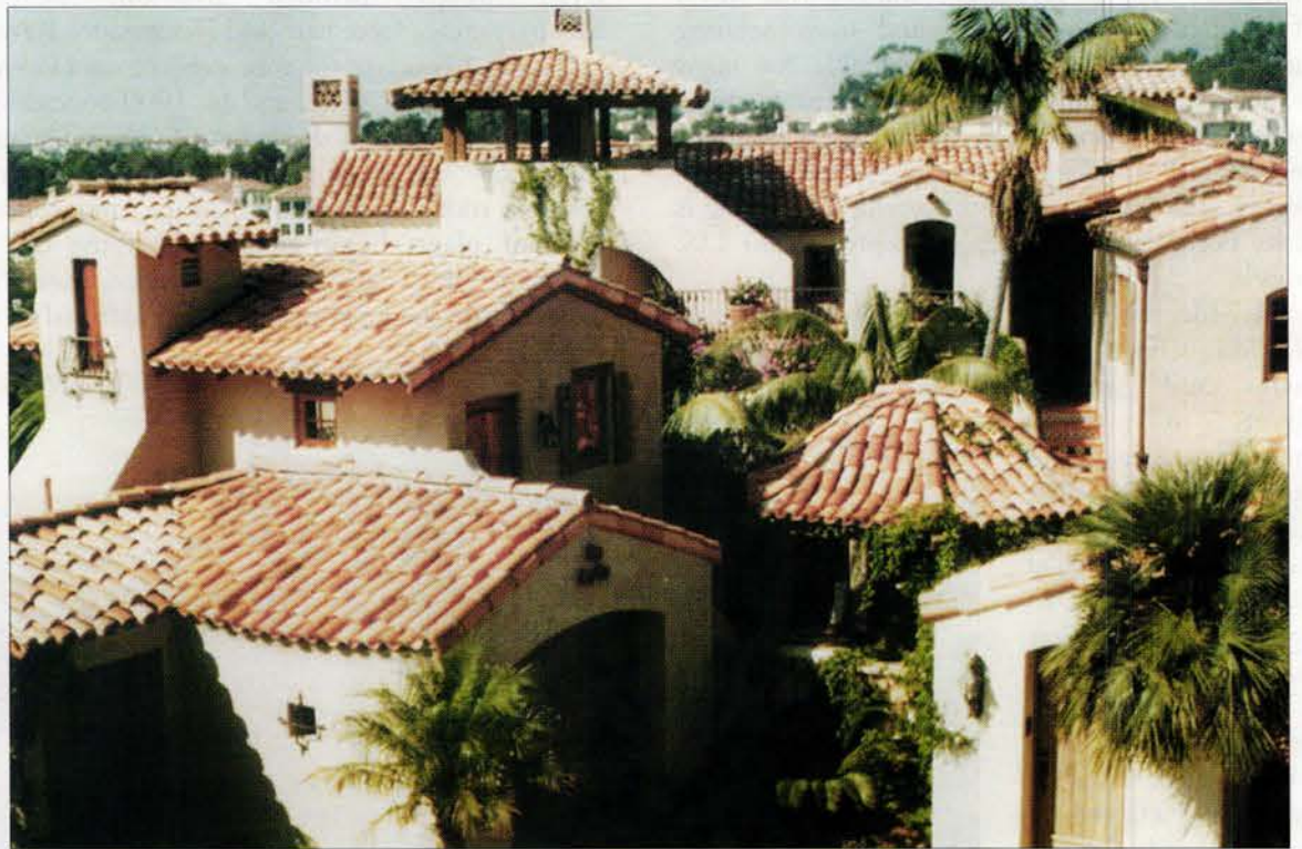
"Spanish tile" has come to mean a one-piece interlocking "S" style with one convex and one almost-flat horizontal surface. The style was introduced by the Padres in California, Florida, and Texas, although it fell out of favor for a while as less expensive substitutes became available. The style has made a rebound, thanks to the popularity of Mission, Spanish, Mediterranean, and Renaissance Revival styles. Shown here is a community topped with Spanish style clay tile roofing supplied by Roof Tile and Slate Co. of Carrollton, Tex.
