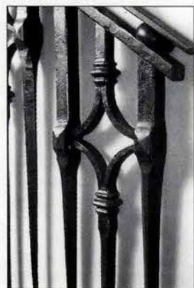
This detail of a fully-forged stair railing, hand-crafted by FINE ARCHITECTURAL METALSMITHS, incorporates 1-1/4-in. pickets tapered to slender octagonal faces, Gothic arches alternating with hot-split terminals, and power-hammered collars. Write in No. 2640
