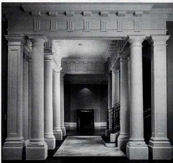
CLASSIC MOULDINGS created these Doric columns, 3/4-square columns with recessed panels, and tri-glyph frieze and cornice, which combine to create a striking residential hallway.
