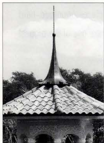
COPPER CRAFTSMAN created this copper steeply pitched roof that sits atop the decorative bell/clock tower of a pool house in Ft. Lauderdale, Fla. Write in No. 746
