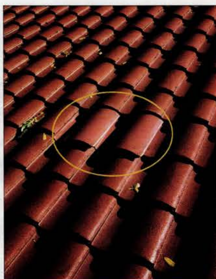
O'HAGIN'S cloaked-vent tiles are used instead of two roof tiles to provide ventilation in a clay or cement tile roof. Write in No. 273
