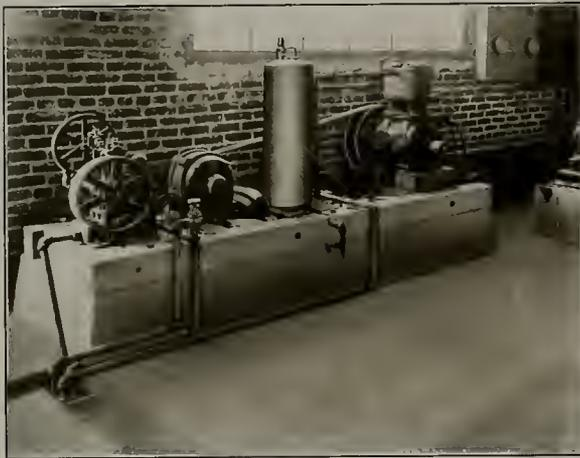
"Hawks" water tube boiler into the distributing mains and system at an initial pressure of 20 pounds per square inch. The city water mains are connected direct to the boiler through a pressure-reducing valve and feed water heater, the latter being a series of coils placed in the pit behind the bridge wall and in the combustion chamber of the fire box.
