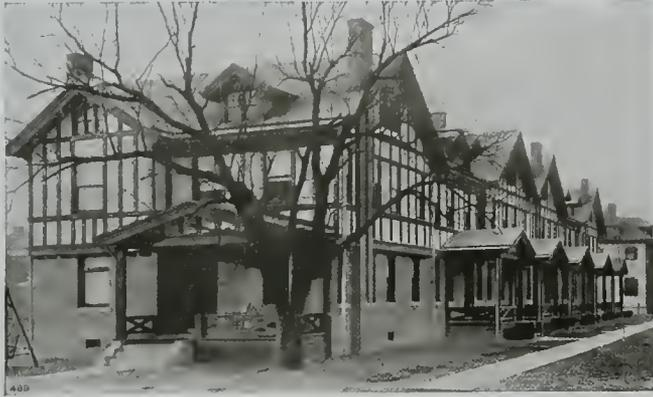
Flat Asbestos Building Lumber Used in Half Timber Effect on Residences
