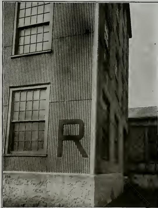
Ambler Corrugated Asbestos Used as Siding with Ambler Flat Asbestos Building Lumber for Framing, and Asbestos Ridges Roll on Corners. Neighboring Building Covered with Century Asbestos Shingles
