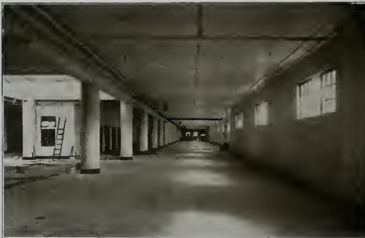
Metal Lath and Plastered Ceiling—Meyer System Floor Construction
