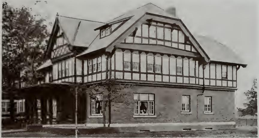
Francis Line Residence, Cleveland, Ohio. J. Milton Dyer and F. G. Bates, Architects. Asbestos "Century" Shingles applied American Method on the Roof and Asbestos Building Lumber on the Sides.
