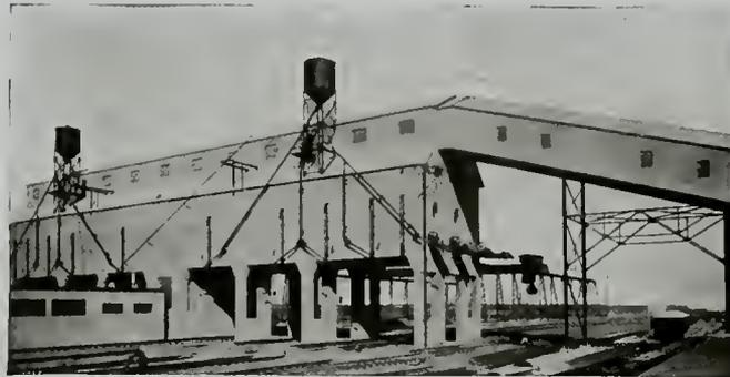
Ambler Corrugated Asbestos Roofing and Siding as Applied to Coal Pockets
