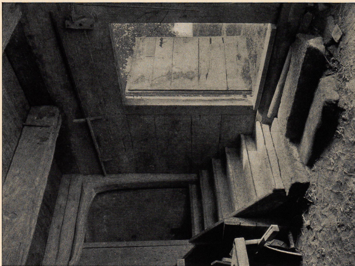
Plank Stairs and Door, Framing, etc. (See Measured Drawing Below) THE MAJOR CHARLES FROST GARRISON HOUSE—1738—EAST ELIOT, MAINE
