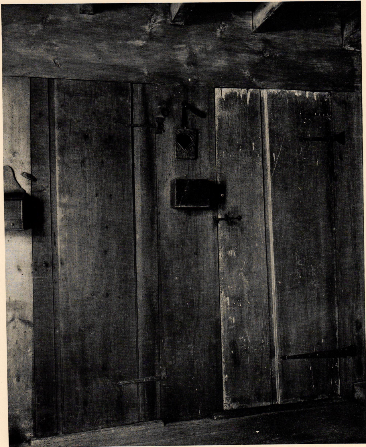
Batten Doors to Kitchen Closet and Entry HASKELL HOUSE, WEST GLOUCESTER, MASSACHUSETTS, 1652
