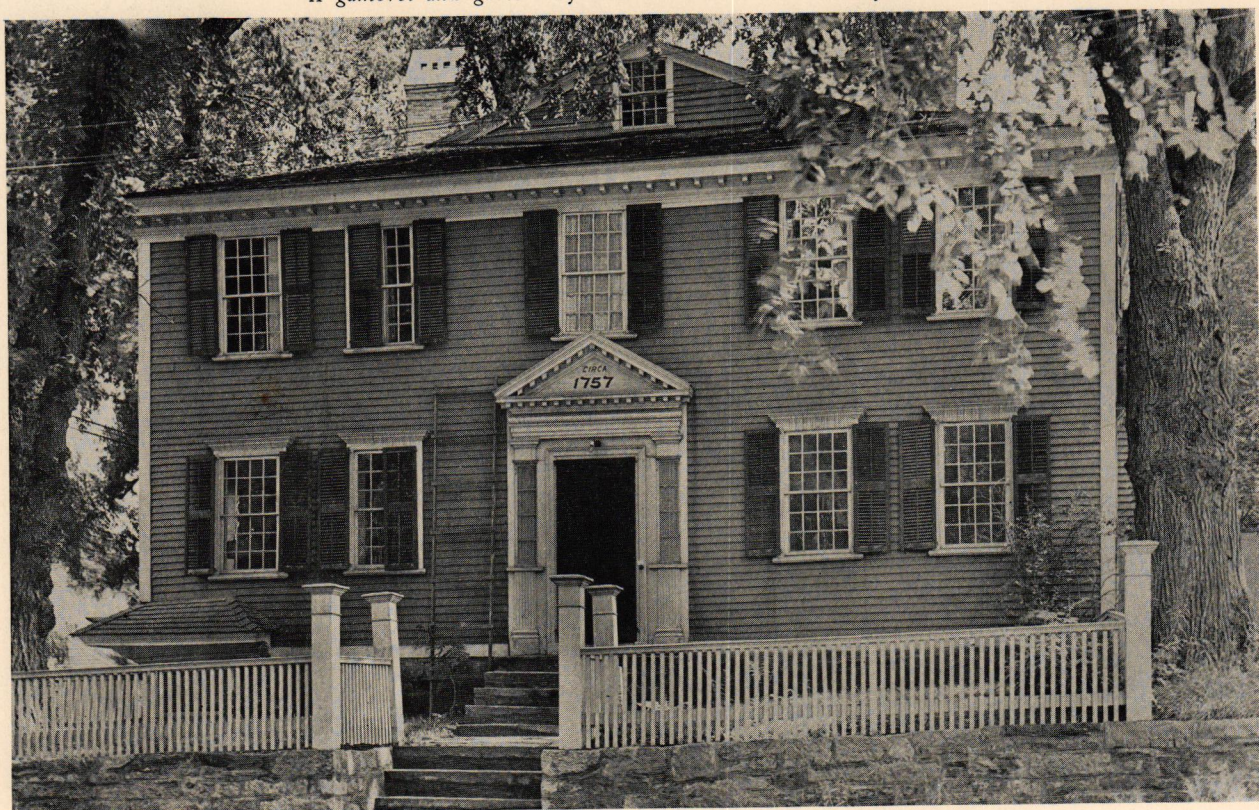
A 1757 HOUSE, EAST GREENWICH, RHODE ISLAND Another example of the gable on hip roof—this time with a window.
