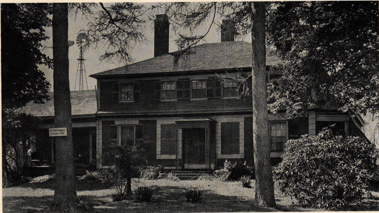
GOVERNOR TRUMBULL HOUSE, LEBANON, CONNECTICUT, BUILT 1753 A hip roof with short ridge.
