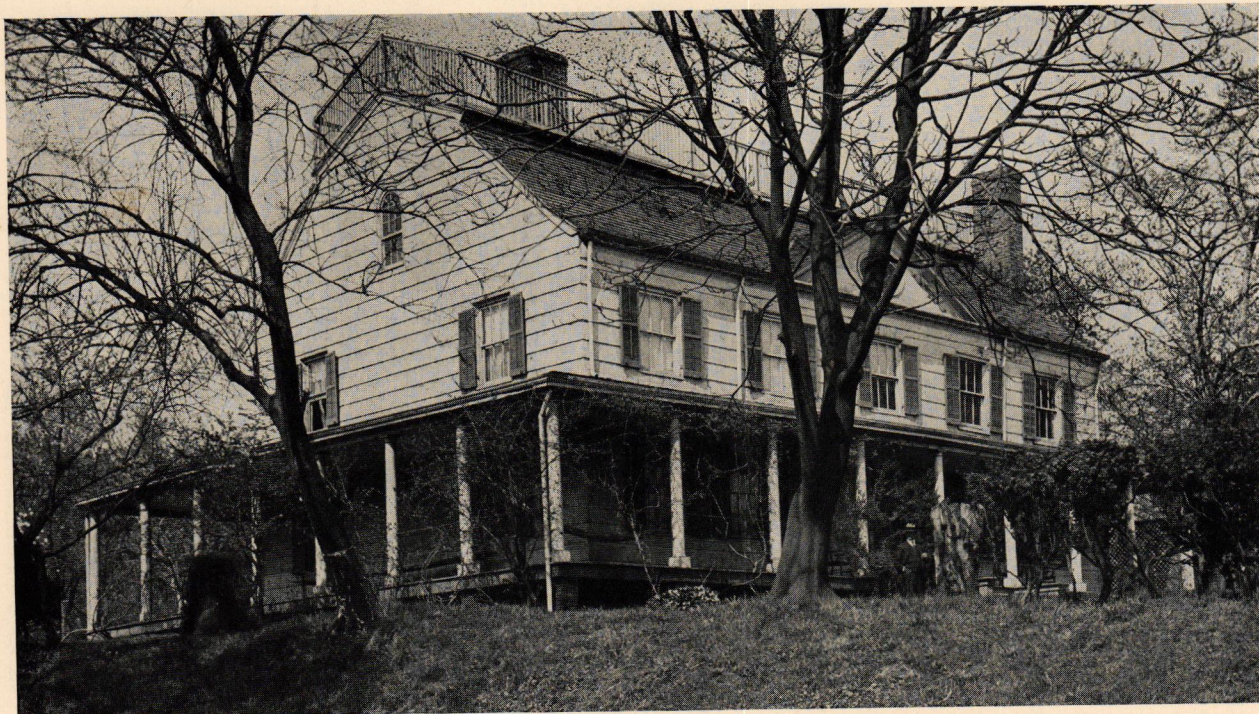
THE PRINCE HOUSE, FLUSHING, NEW YORK A gambrel and gable roof used on a late 18th Century house.
