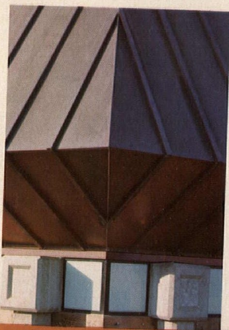
New Field House, University of California at Santa Cruz. Copper encloses the terminal chords of the two-way steel truss that spans the large main area of the building. Repetition of copper above an open stairway unites the design. The unusually prominent drip created at the eave gives strong definition to the roof.
