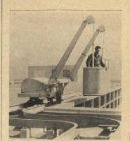
**Building maintenance.** Oneman window-washing scaffold is roof-mounted, and moves vertically, horizontally, and toward or away from the building face. Movement is controlled electrically by the operator. Electrical conductors are encased in steel hoisting cable, thus eliminating separate control cables. Lifting speed is 40 fpm; and horizontal speed is 48 fpm. Patent Scaffolding Co., Div. of Harsco Corp., 38–21 12 St., Long Island City, N.Y. 11101. *Circle 118, Readers' Service Card*
