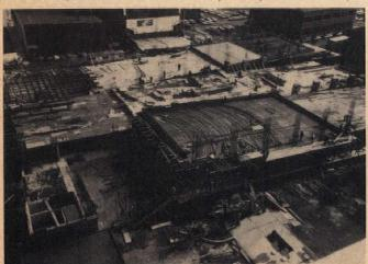
Tendons have been uncoiled on slab forms in foreground; in upper right, part of the concrete placement has been completed with additional concrete being pumped into place.
